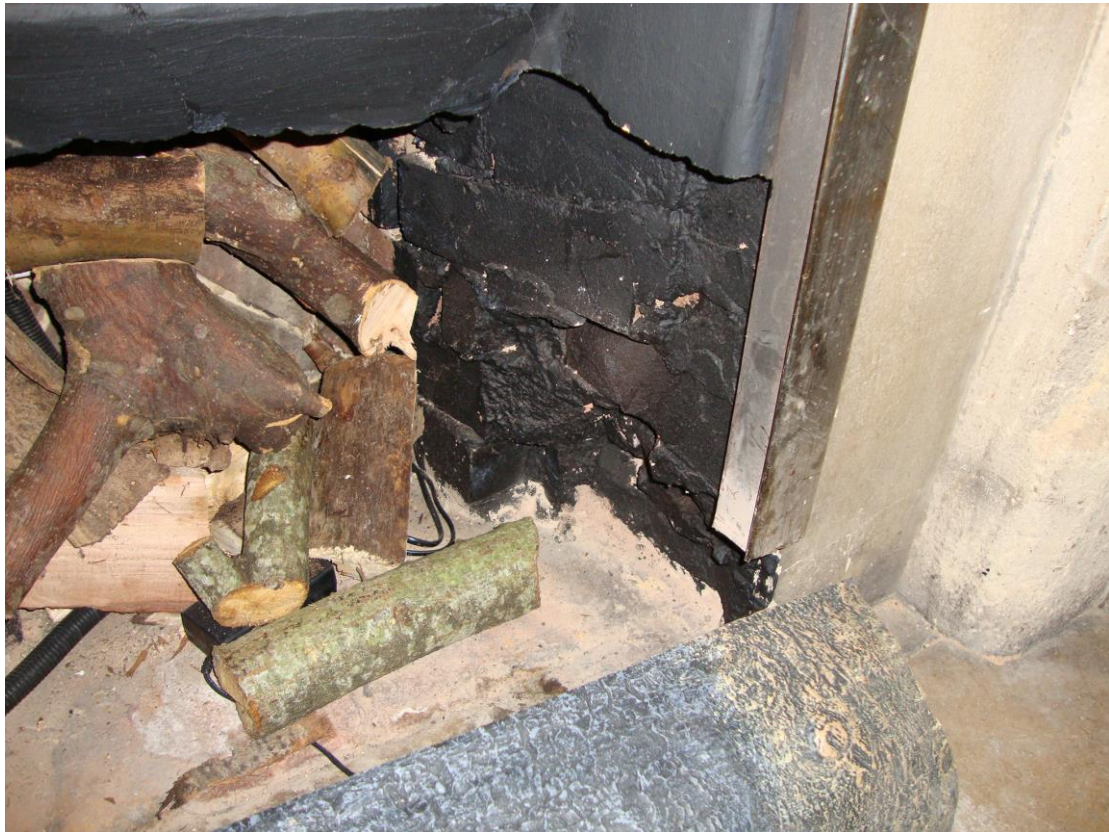
2.6 EXISTING FIREPLACE SHOWING MODIFICATIONS TO HEARTH (RHS)
