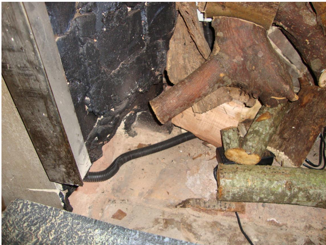
2.5 EXISTING FIREPLACE SHOWING MODIFICATIONS TO HEARTH (LHS)
