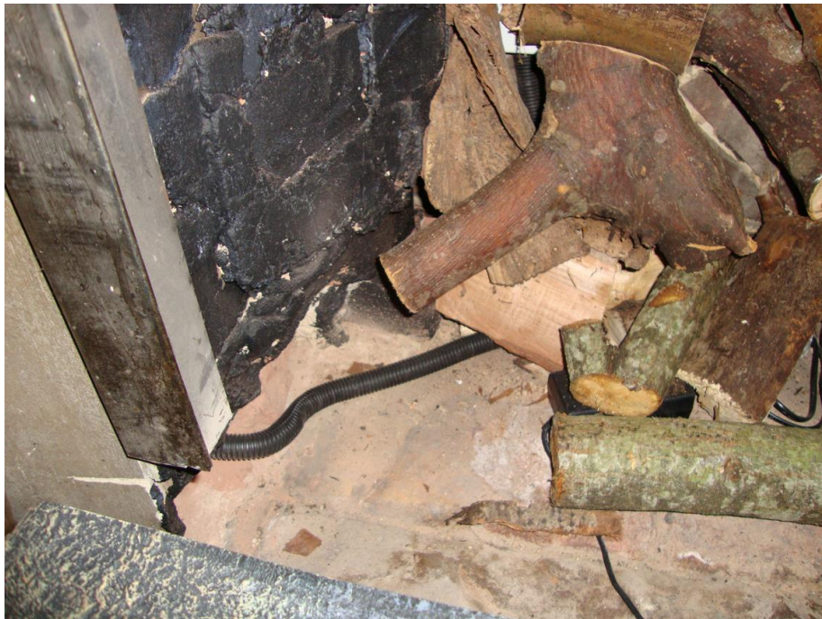
5.09 Junction between brickwork enclosure and hearth showing modification and route of gas supply.
