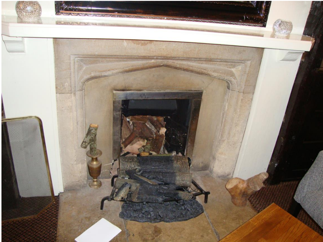
2.4 EXISTING FIREPLACE SHOWING NEW GAS FIRE
