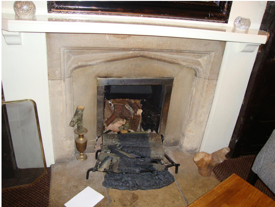
5.08 Existing Fireplace and surround
