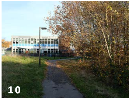
At the western end of the site looking back (east) towards the school building
