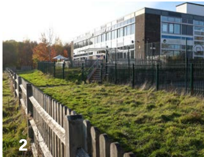
2 Existing school building (southern elevation) looking west
