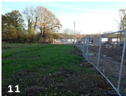
Western end of the site and initial works for access to the strategic Woodcroft Farm site
