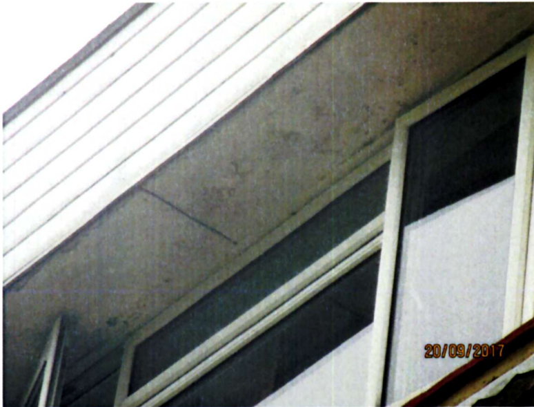
Photo 3 - Existing Facia Board and Soffit
