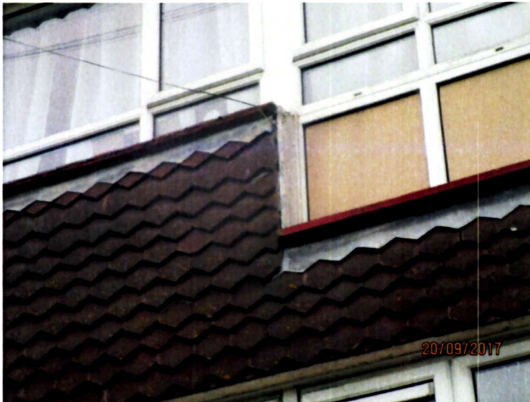
Photo 4 - Tile hanging to front elevation
