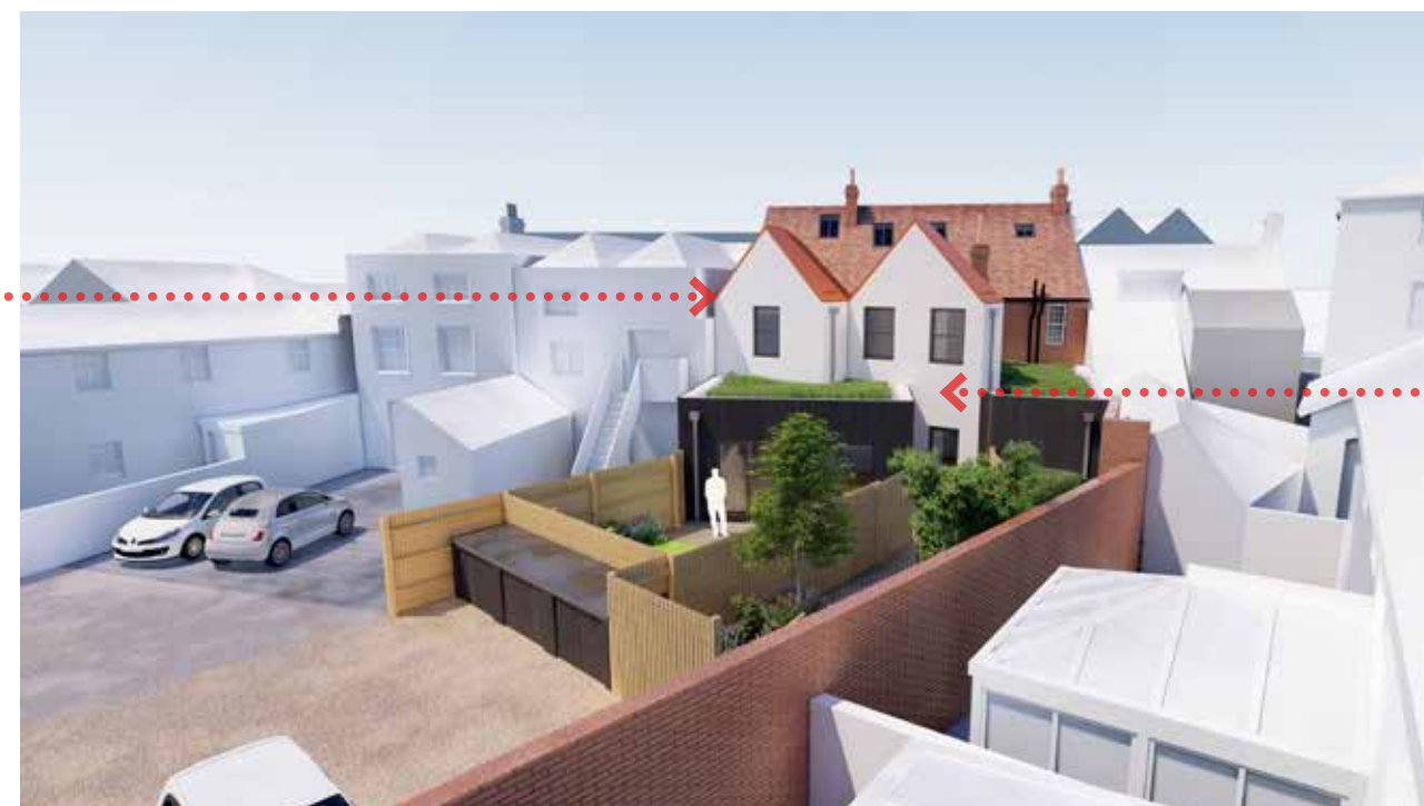
aerial view of rear elevation and courtyard
