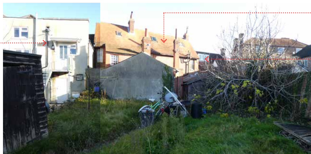
View looking towards rear elevation of property
