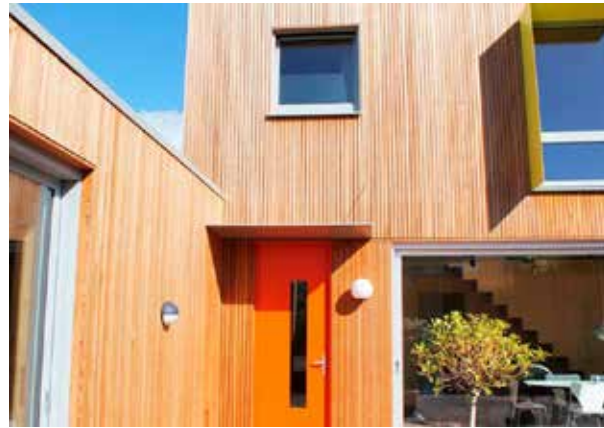
Hampshire Passivhaus, Convent Lane, Emsworth http://www.ruthbutlerarchitects.com
