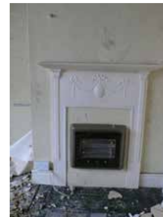
Chimney breast and fire place to first floor eastern boundary room
