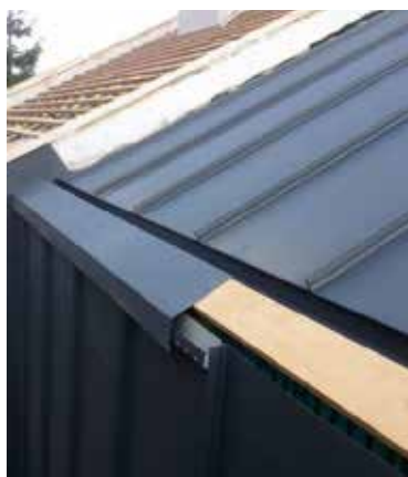
metal standing seam roof with hidden gutter
