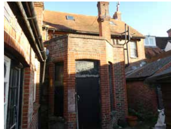
Looking towards rear elevation of property
