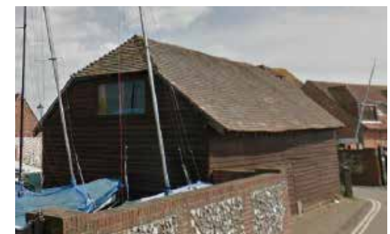
Sailing Club storage barn, Bridgefoot Path, Emsworth http://www.google.co.uk
