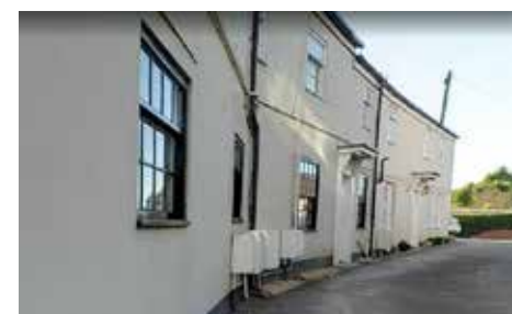
LOCAL VERNACULAR AND DETAILING IN WEST STREET, EMSWORTH
