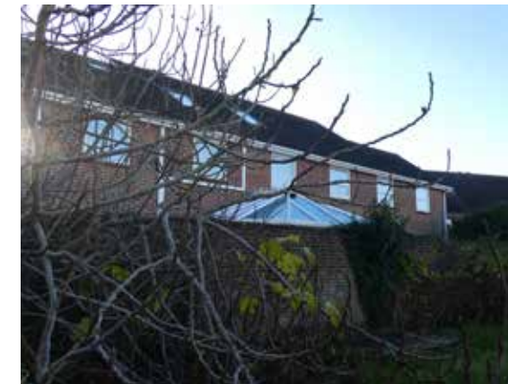
Rear elevations of 1D and 1E School Lane; conservatory on the ground floor and rooflights
