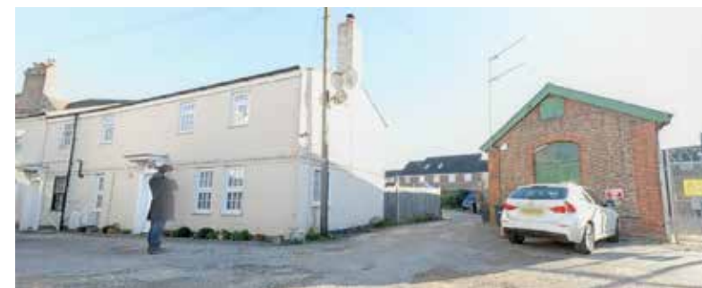
COTTAGES IN THE VICINITY OF 2 WEST STREET, EMSWORTH
