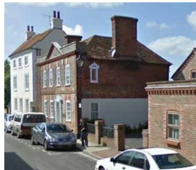
LOCAL VERNACULAR AND DETAILING IN WEST STREET, EMSWORTH
