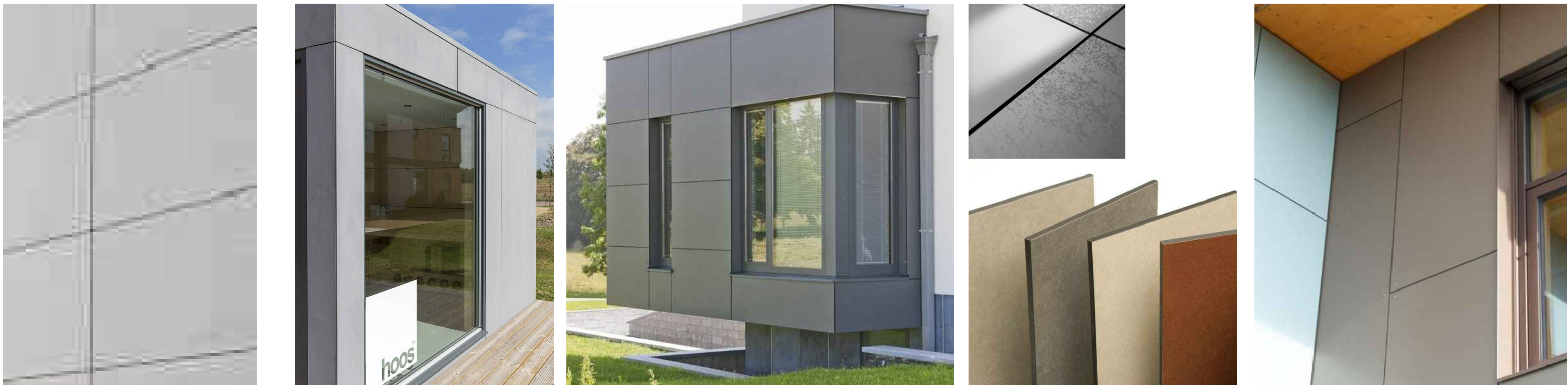
EXAMPLE OF TRESPA AND ETERNIT CLADDING PANELS
