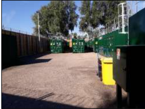
Figure 1: Hardstanding within generator compound
