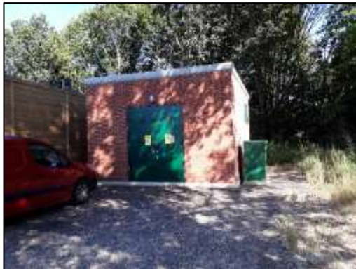
Figure 3: Flat roof building
