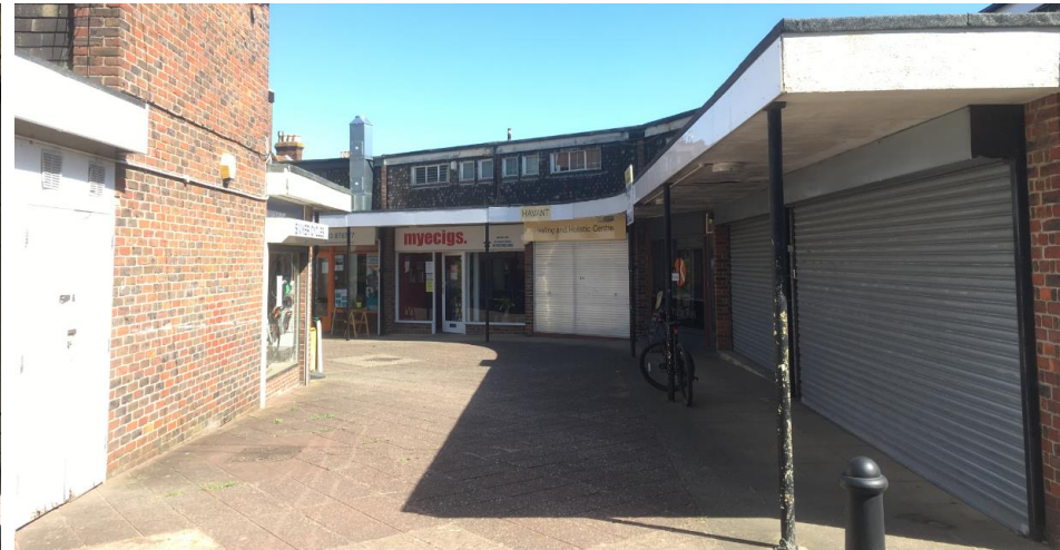
Figure 5 View North into Arcade from Footpath Link
