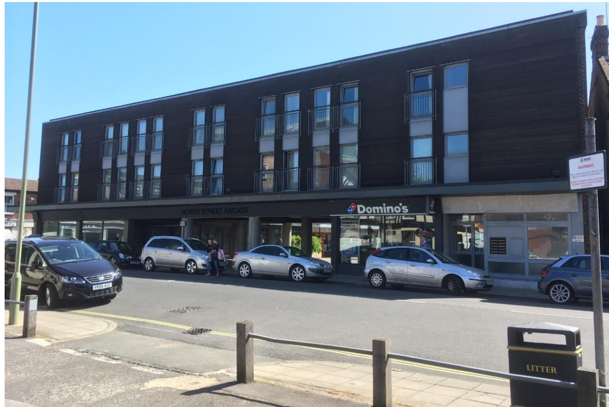
Figure 3 View of North Street Arcade from West side of North Street
