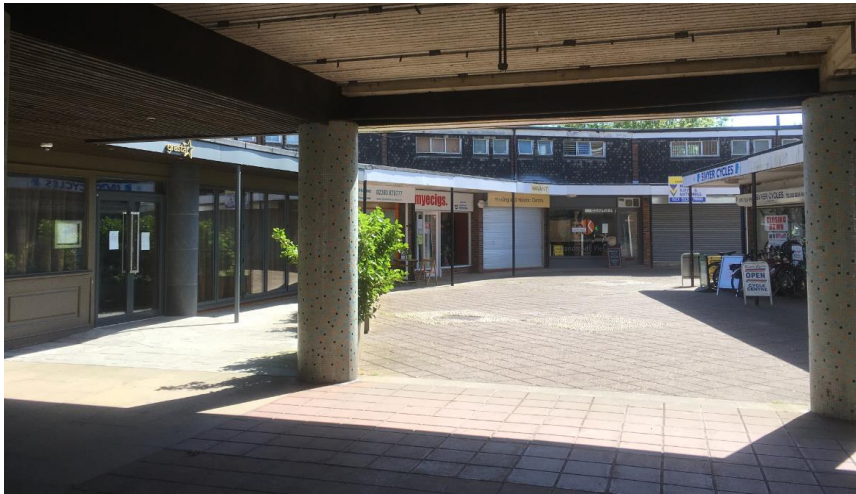
Figure 4 View East Through Undercroft from North Street
