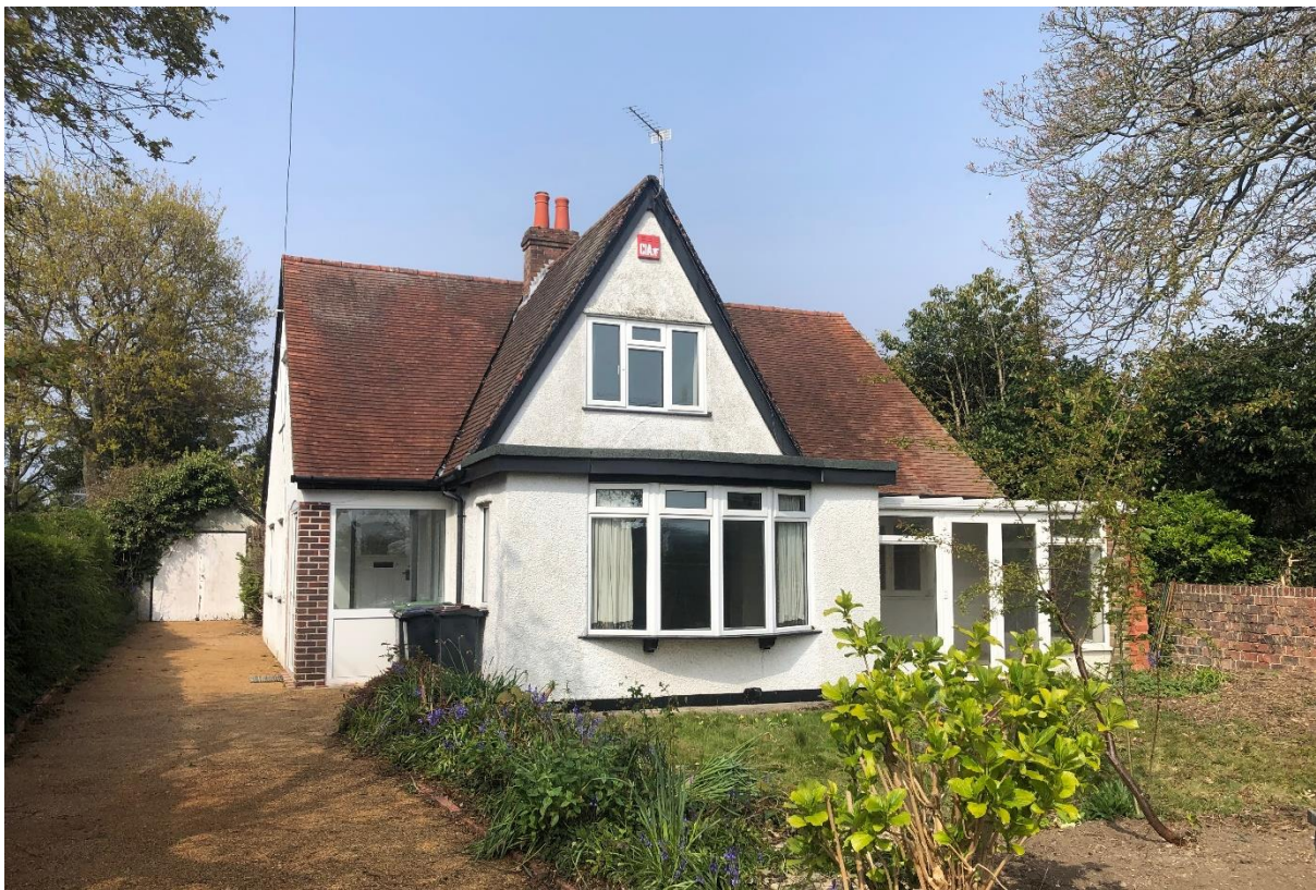
Figure 1: Front Elevation of 61 Warblington Road
