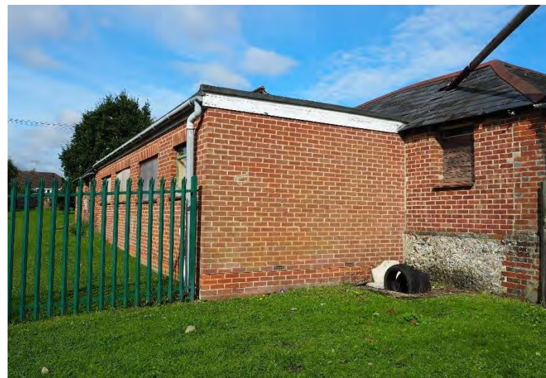
Plate 62: Modern extensions to the south of Building 6.
