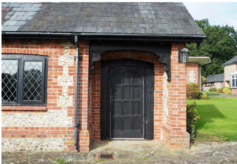
Plate 28: Northern porch to Building 3.
