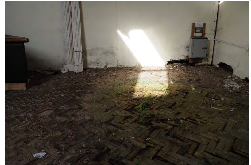
Plate 67: Flooring in Building 8.
