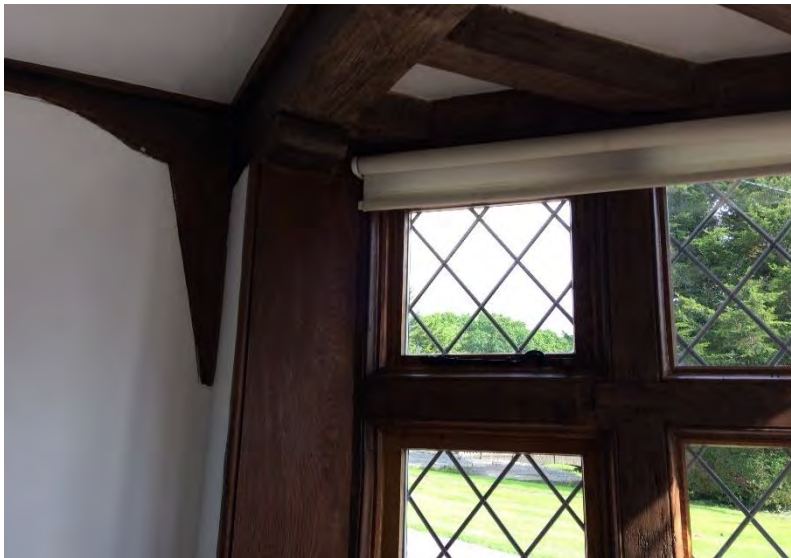
Plate 38: Detail of wooden window frames.
