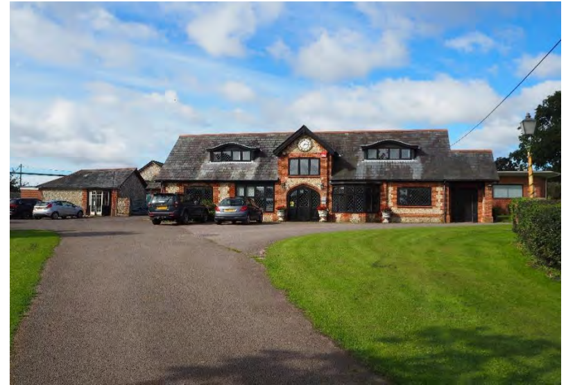
Plate 26: East elevation of Building 3.
