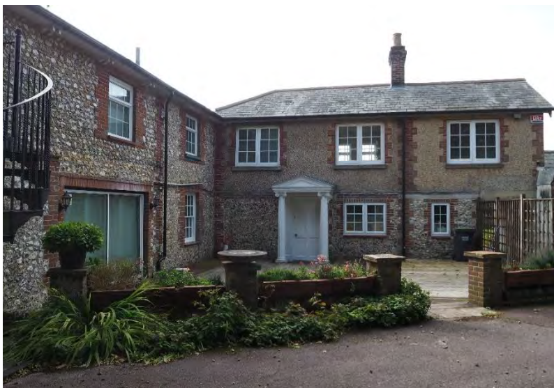
Plate 21: North elevation of the rear range of Building 1.
