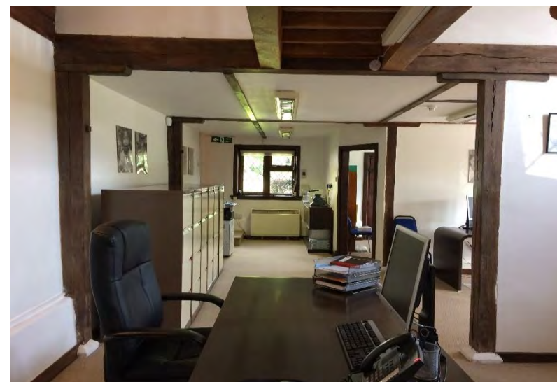
Plate 33: View north on the ground floor of Building 3.
