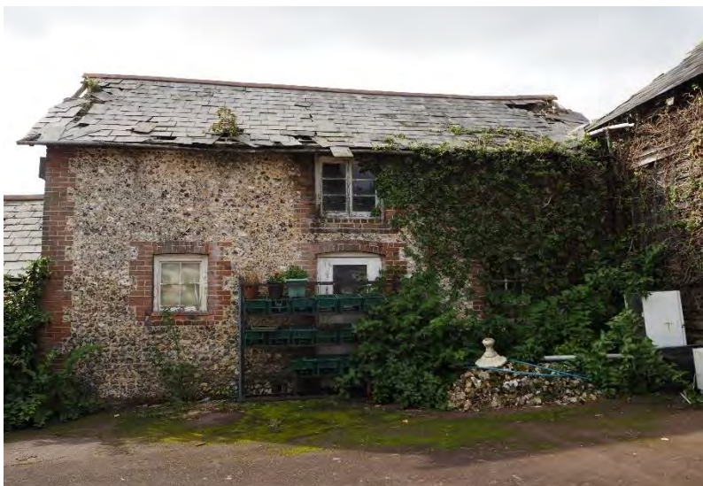
Plate 60: North elevation of the 2 storey element of Building 6.
