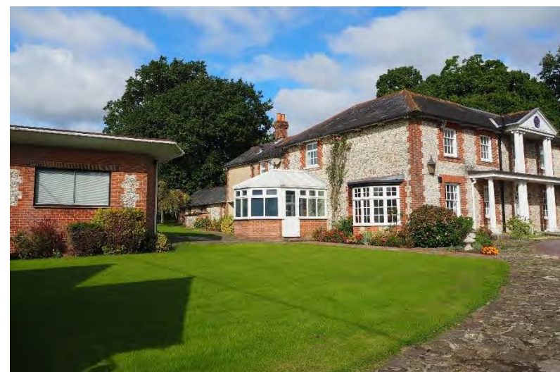
Plate 20: Later extensions on the south elevation of Building 1.
