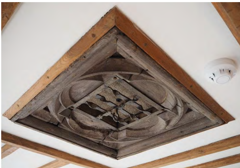
Plate 44: Detail of wooden carved rose in the ceiling of Building 3.
