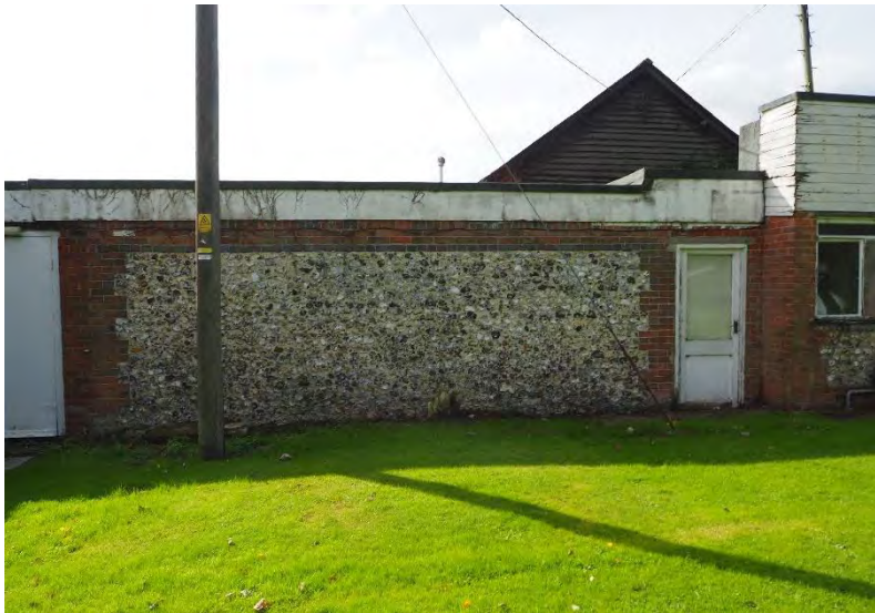
Plate 46: Western end of the north elevation of Building 4.
