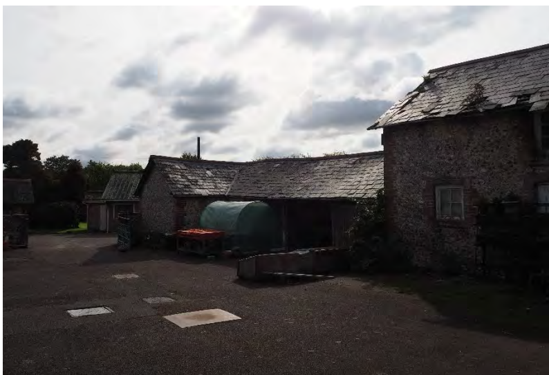
Plate 61: North elevation of Building 6.
