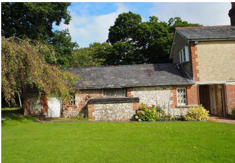
Plate 23: South elevation of Building 2.
