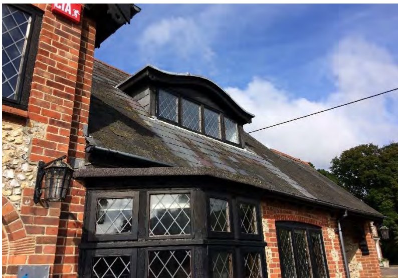
Plate 31: Detail of fenestration openings on the north elevation of Building 3.
