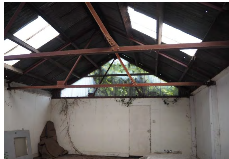
Plate 65: View south within Building 7.
