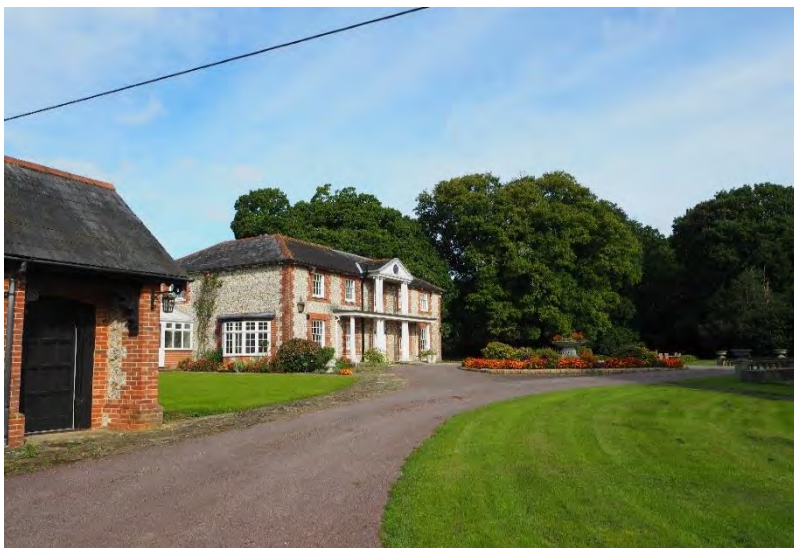
Plate 4: View north across the Site.
