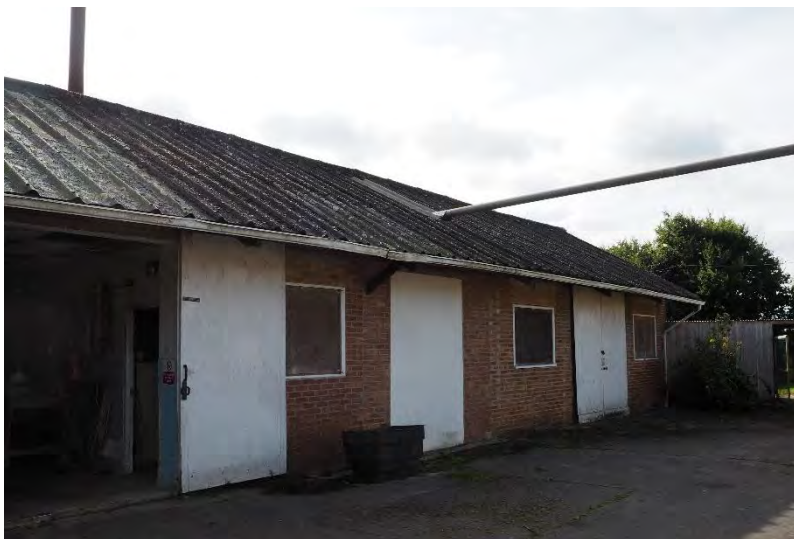
Plate 71: West elevation of Building 10.
