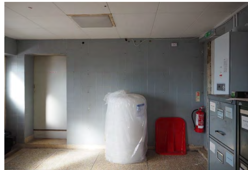
Plate 52: Interior of the central elements of Building 4.
