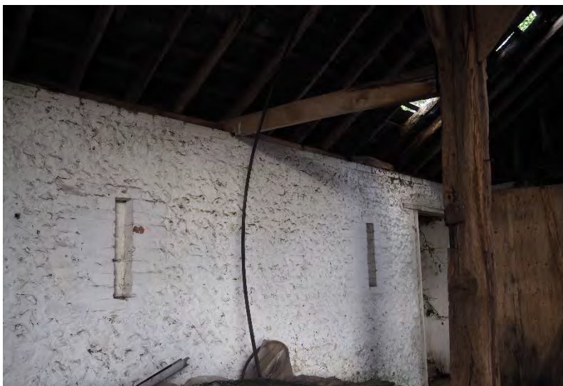
Plate 58: West elevation of Building 5.
