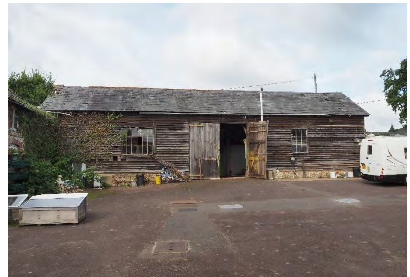
Plate 53: East elevation of Building 5.
