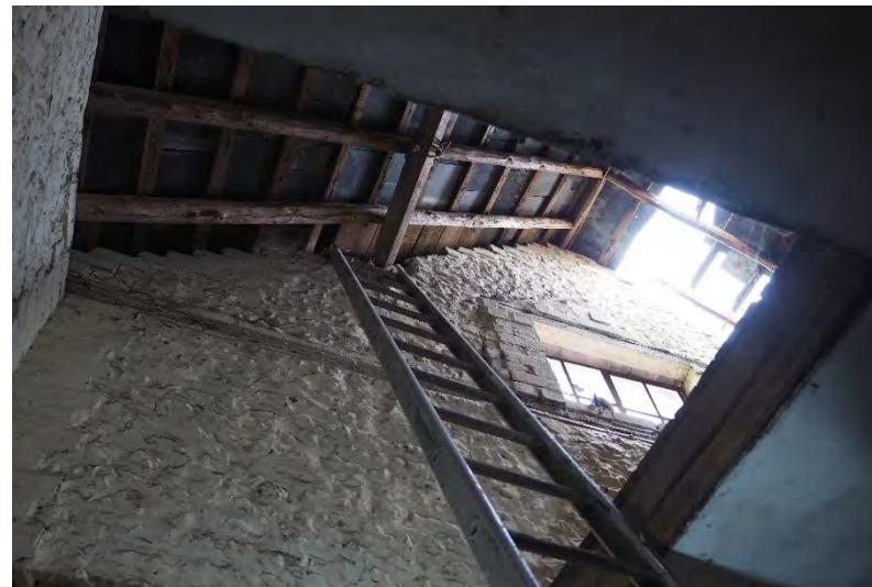
Plate 63: Interior of the 2 storey element of Building 6.
