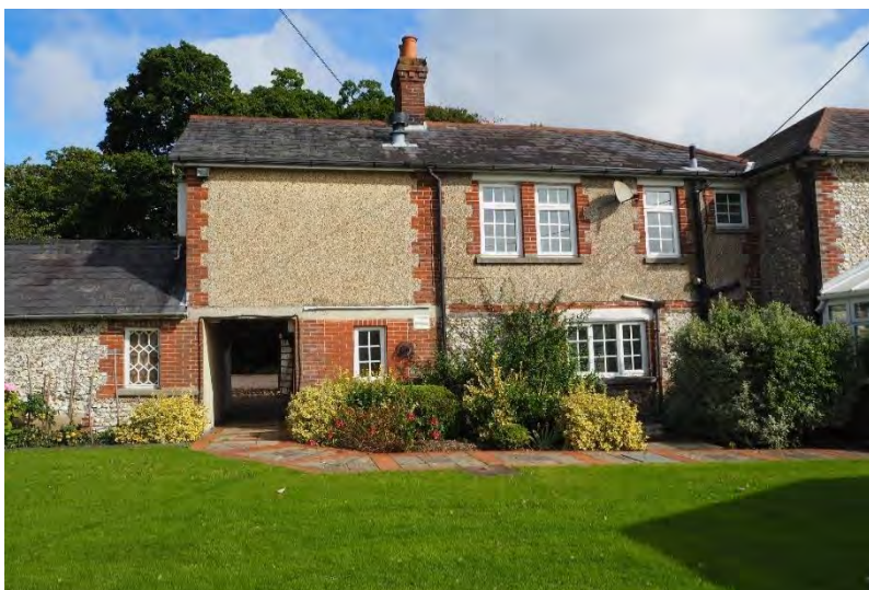
Plate 22: South elevation of the rear range of Building 1.
