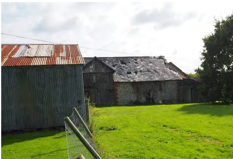
Plate 54: West elevation of Building 5.
