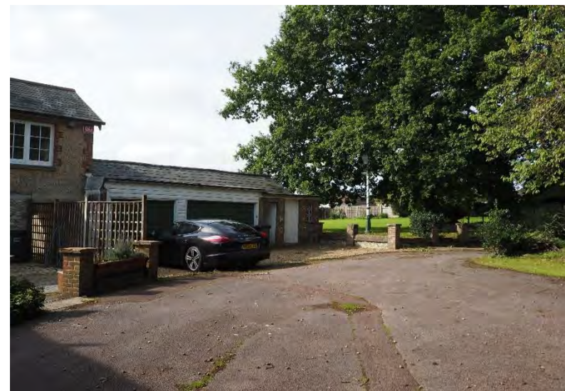
Plate 24: North elevation of Building 2.
