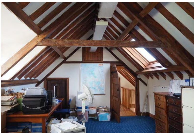
Plate 35: Detail of roof structure in Building 3.
