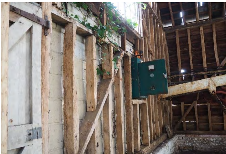
Plate 59: North elevation of Building 5.
