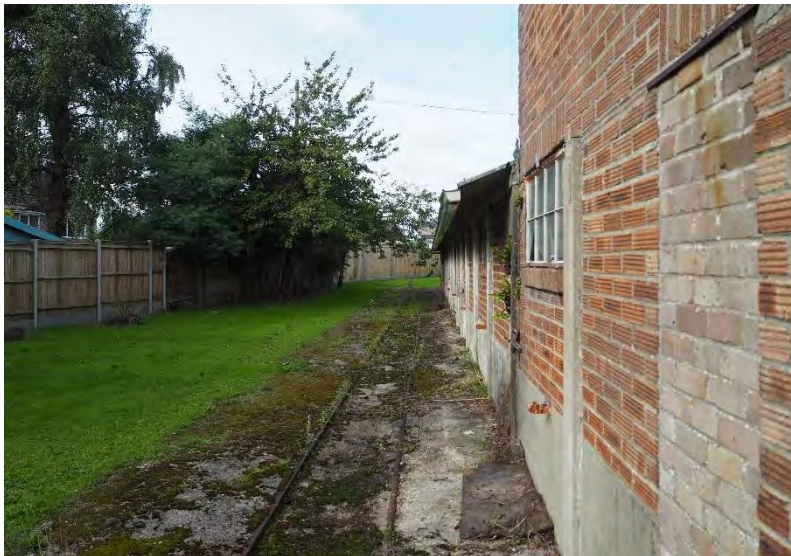
Plate 69: South elevation of Building 9.
