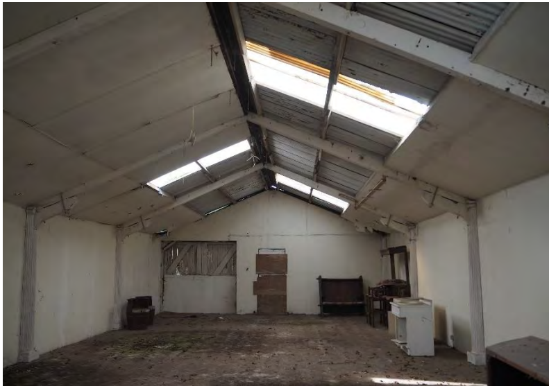
Plate 66: View north within Building 8.
