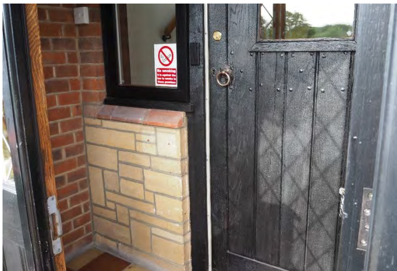
Plate 27: Modern fabric in central entrance to Building 3.
