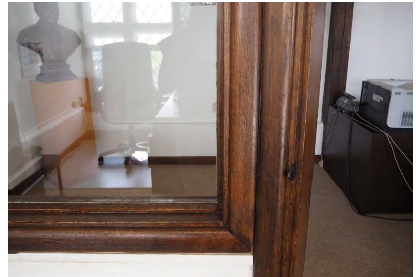
Plate 39: Detail of partitions on the ground floor of Building 3.
