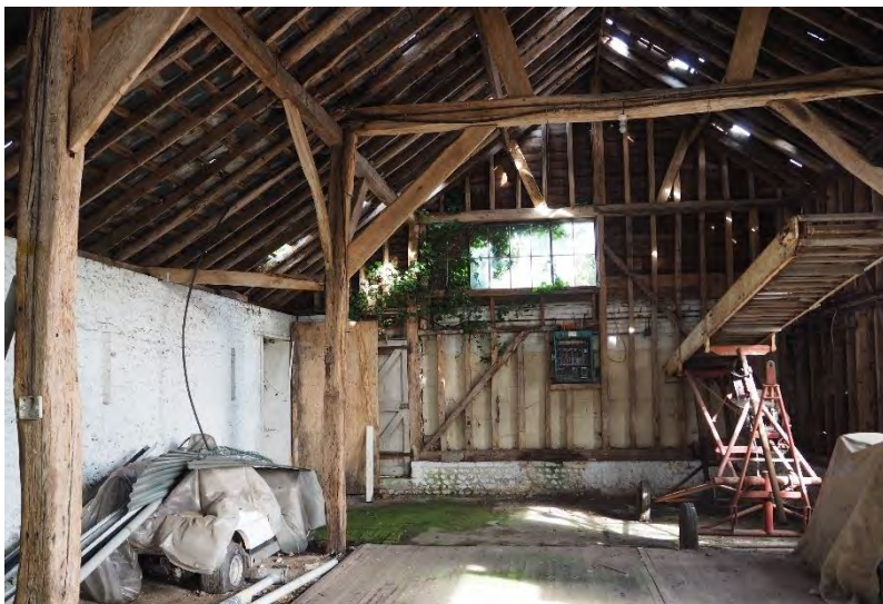
Plate 55: View north in the interior of Building 5.
