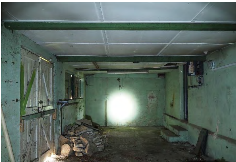
Plate 64: Interior of modern elements of Building 6.
