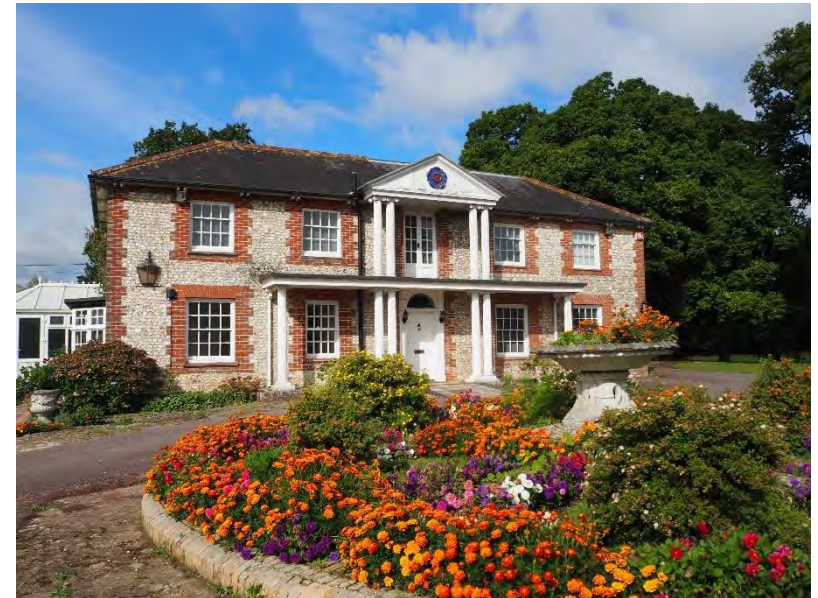
Plate 18: Principal, east, elevation of Building 1.
