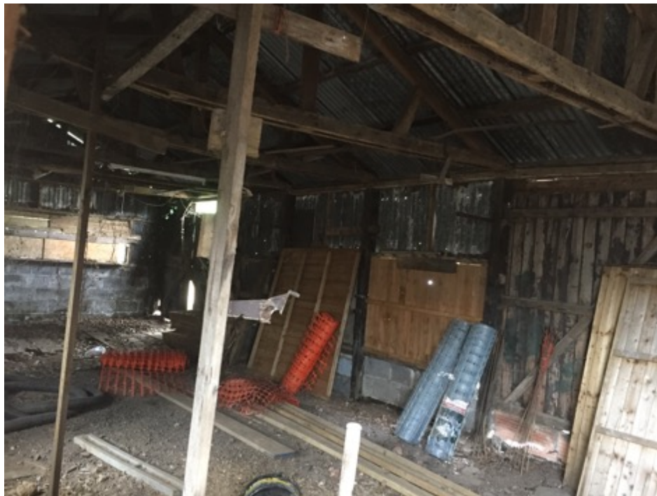
Photograph 4 Interior of the building in the centre of the site, showing storage of building materials, fencing and wooden fence panels.
