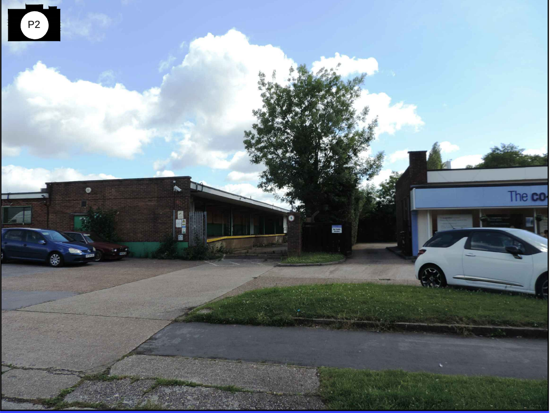
View of the western aspect of the building, the low quality ash tree (T3) is prominent only as a result of the absence of other trees but is unsustainable due to its structural condition and location.
