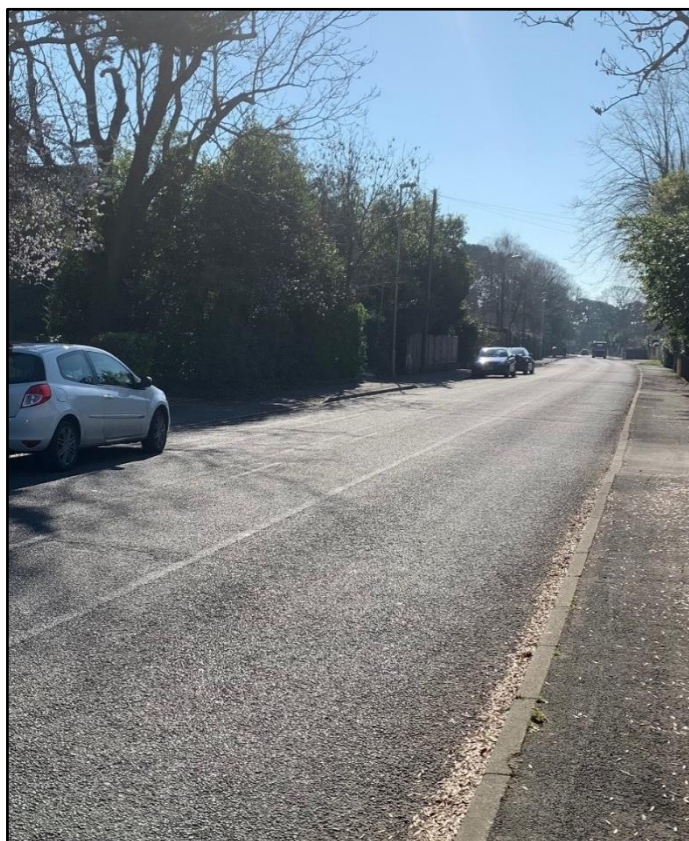
Figure 2.1 – New Brighton Road Towards the South
