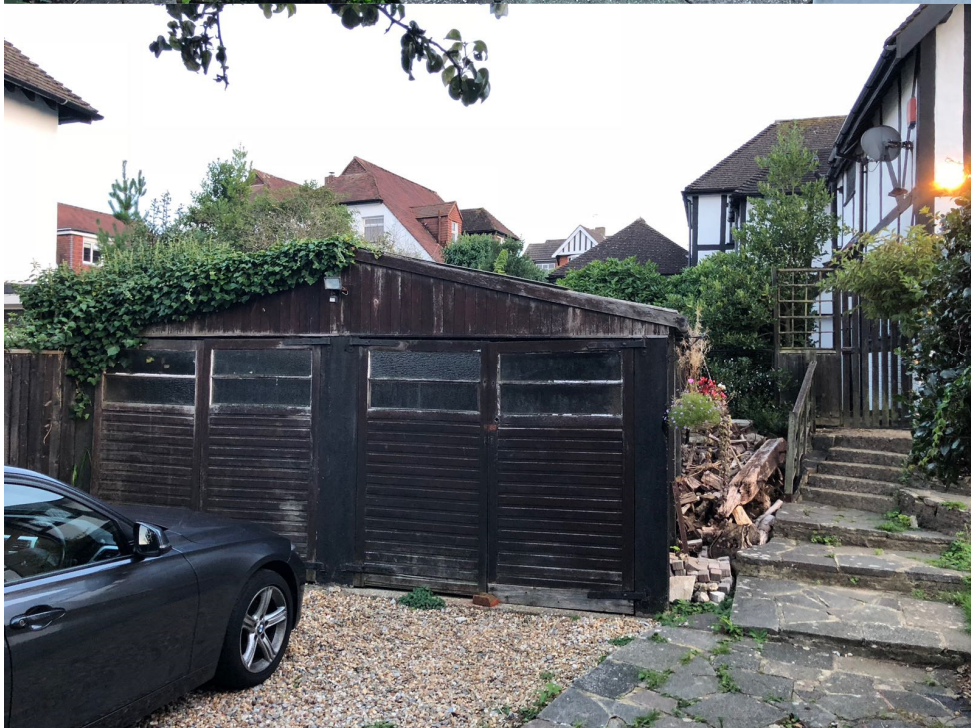
View of driveway back to the existing dilapidated garage.
