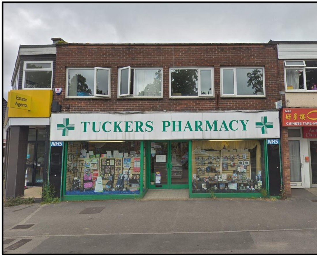
Photo 1.1 – Existing shopfront to Tuckers Pharmacy, Cowplain
