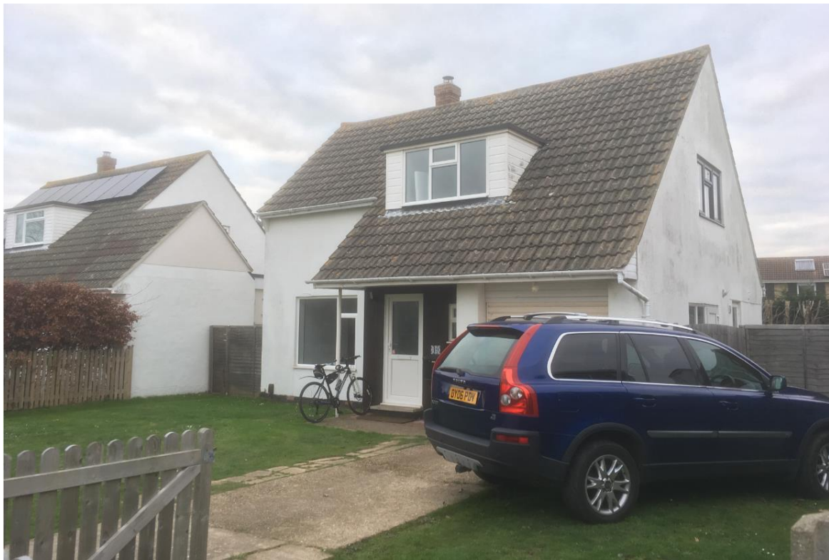
Figure 8 Photo of 49 St Thomas Avenue
