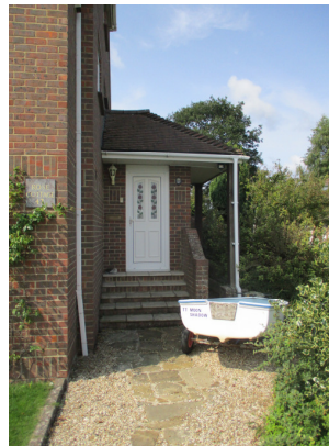
Fig 4 - View of the existing entrance into the property along the northern side elevation, currently blocking access to the rear garage
