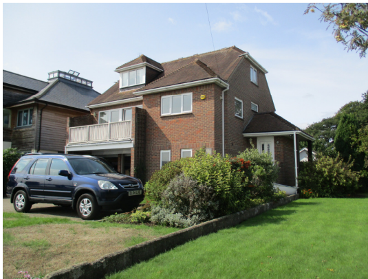
Fig 3 – View of the front of the property from Bath Road showing the existing main entrance into the property along the northern side elevation
