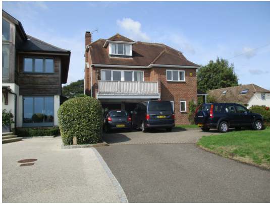
Fig 1 – View of the front of the property showing the existing driveway shared with No.48
