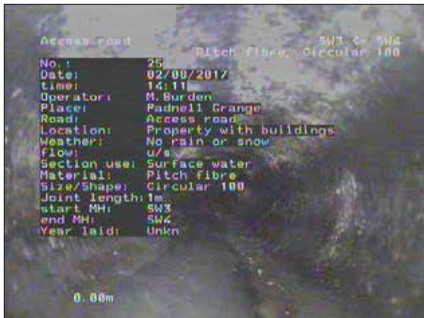
Photo: 184_1a, 00:00:00 0m, Start node type, manhole, reference number: SW3
