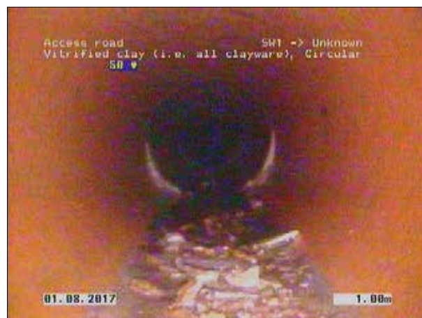
Photo: 69_6a 1m, Survey abandoned, Remark: to much debris in line
