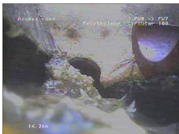
Photo: 135_4a, 00:00:00 14.26m, Finish node type, manhole, reference number: FW7
