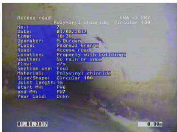
Photo: 7_1a 0m, Start node type, manhole, reference number: FW6
