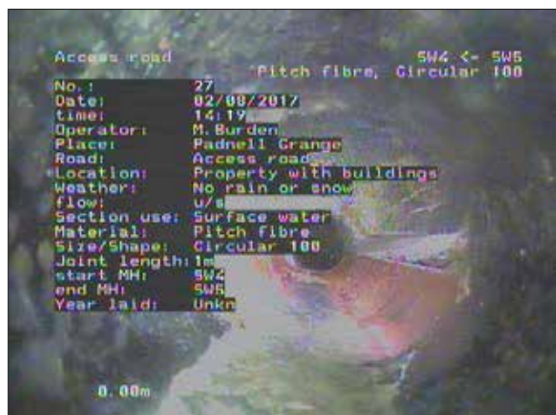
Photo: 192_1a, 00:00:00 0m, Start node type, manhole, reference number: SW4
