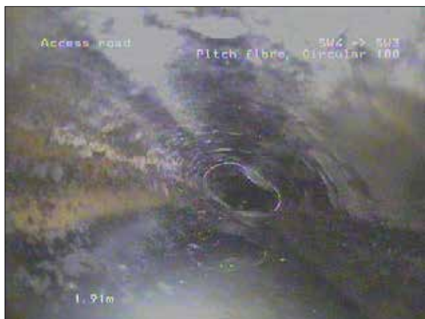
Photo: 191_4a, 00:00:00 1.91m, Survey abandoned, Remark: squashed Pitch fiber line
