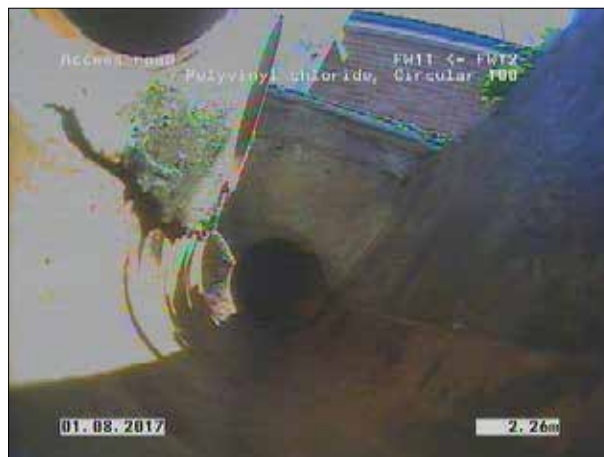
Photo: 63_3a 2.26m, Finish node type, manhole, reference number: FW12
