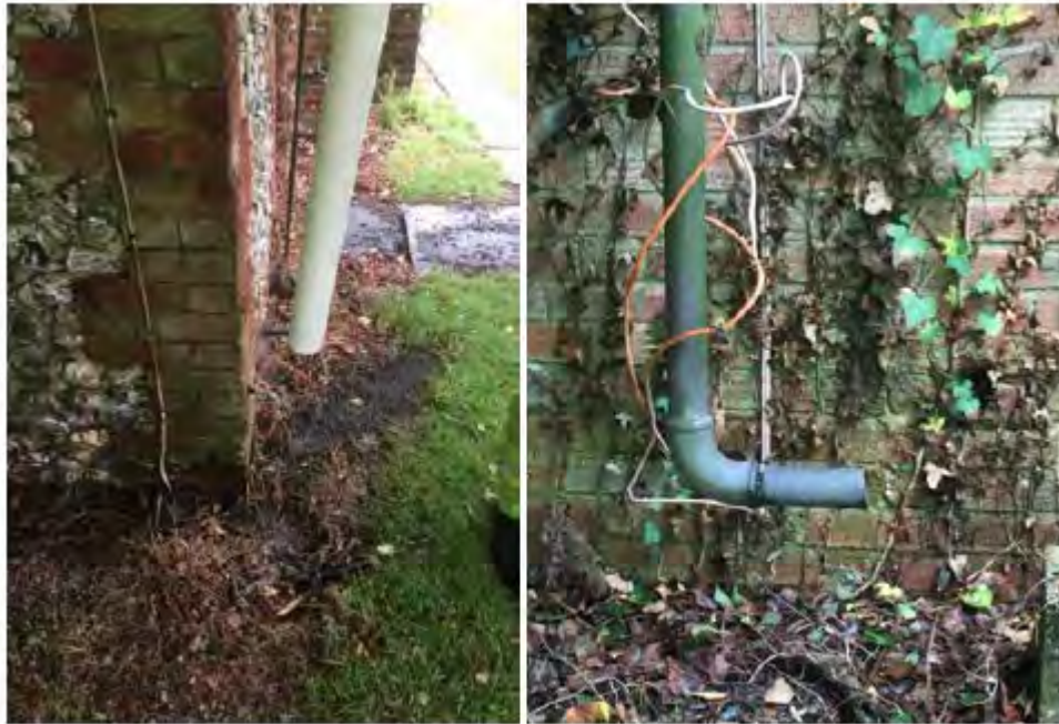
Figure 5.1: Existing Down Pipes
