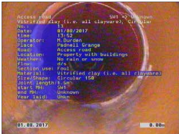
Photo: 74_1a 0m, Start node type, catchpit, reference number: SW1
