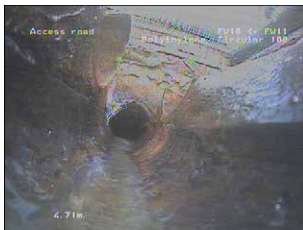
Photo: 24_8a, 00:00:00 4.71m, Finish node type, manhole, reference number: FW11
