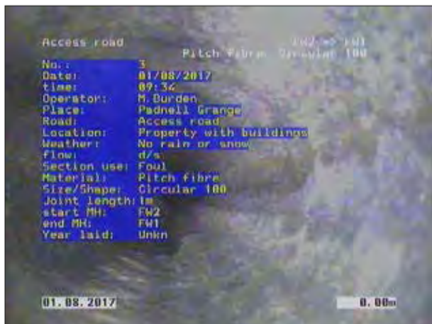
Photo: 19_1a 0m, Start node type, manhole, reference number: FW2
