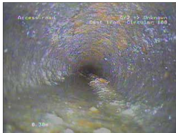
Photo: 123_3a, 00:00:00 0.3m, Settled deposits fine 10 % cross-sectional area loss
