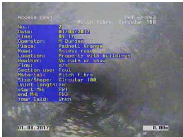
Photo: 11_1a 0m, Start node type, manhole, reference number: FW1
