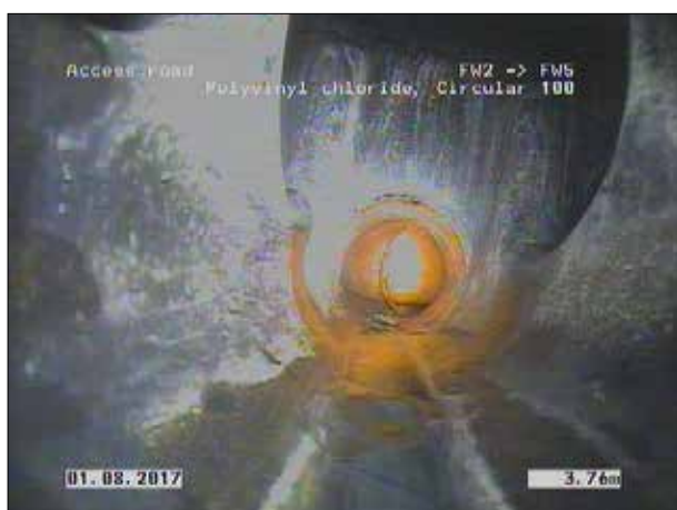
Photo: 4_4a 3.76m, Finish node type, manhole, reference number: FW5
