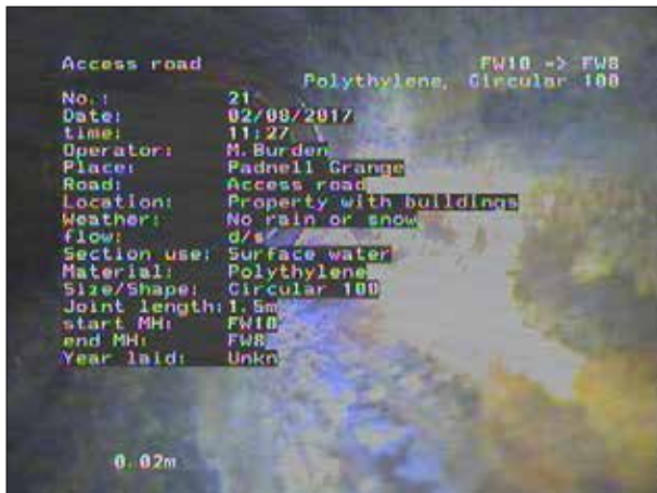
Photo: 147_1a, 00:00:00 0m, Start node type, manhole, reference number: FW10
