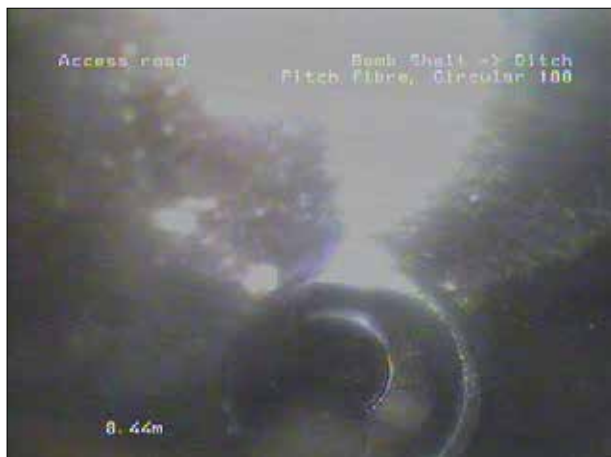
Photo: 215_6a, 00:00:00 8.4m, Junction at 03 o'clock dia 100 mm
