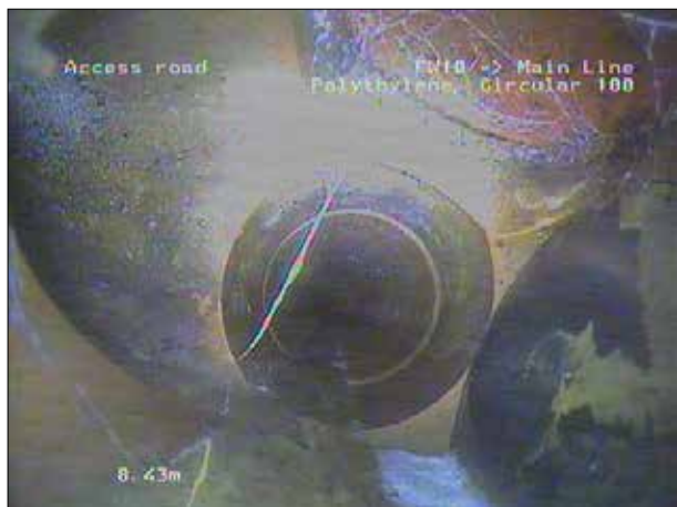
Photo: 152_6a, 00:00:00 8.43m, Junction at 09 o'clock dia 100 mm
