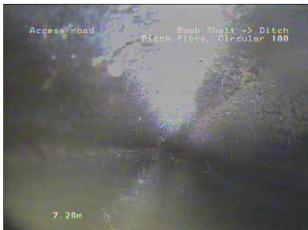
Photo: 31_6a, 00:00:00 7.28m, Water level 15 % height/diameter
