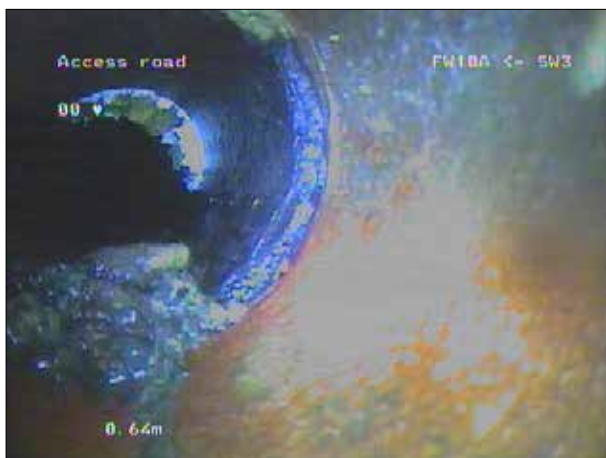
Photo: 173_4a, 00:00:00 0.62m, Settled deposits fine 10 % cross-sectional area loss
