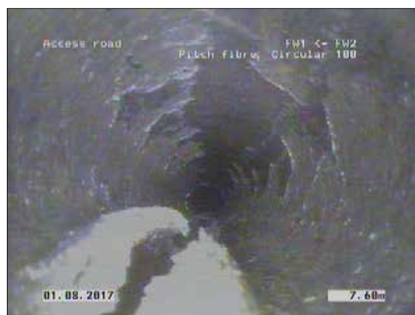
Photo: 1_9a 7.6m, Survey abandoned, Remark: to much scale in line
