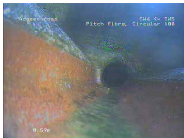
Photo: 194_3a, 00:00:00 0.57m, Finish node type, manhole, reference number: SW5
