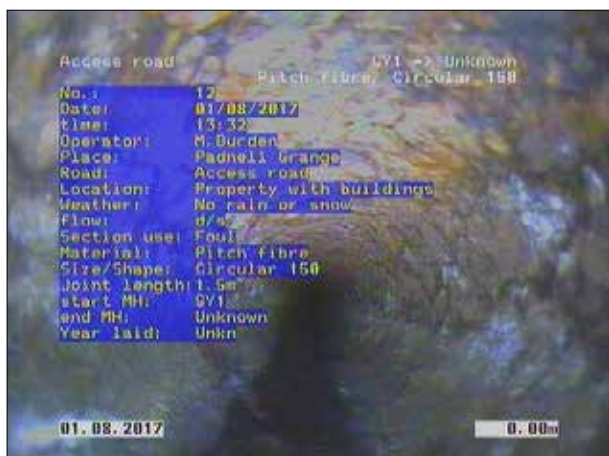
Photo: 70_1a 0m, Start node type, gully, reference number: GY1
