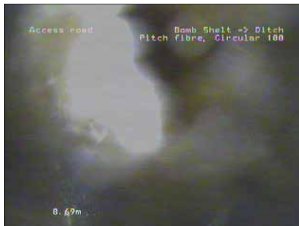
Photo: 31_7a, 00:00:00 8.69m, Survey abandoned, Remark: to much debris in line
