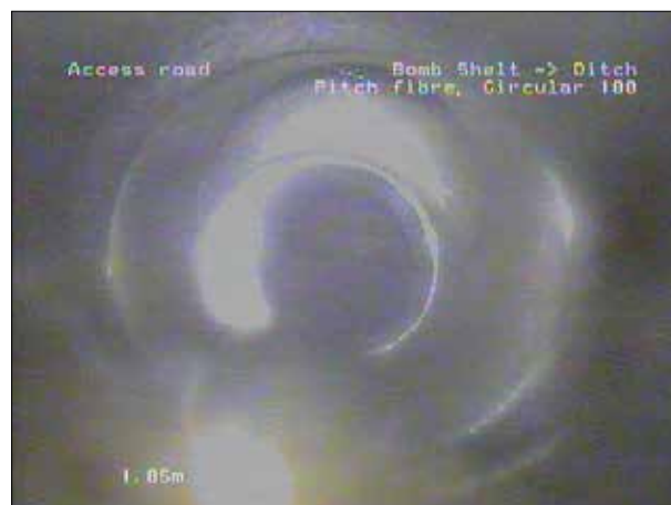
Photo: 212_3a, 00:00:00 1.85m, Junction at 12 o'clock dia 100 mm
