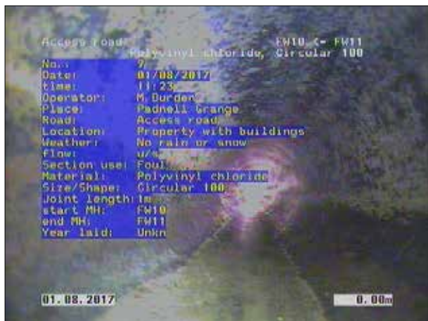
Photo: 58_1a 0m, Start node type, manhole, reference number: FW10
