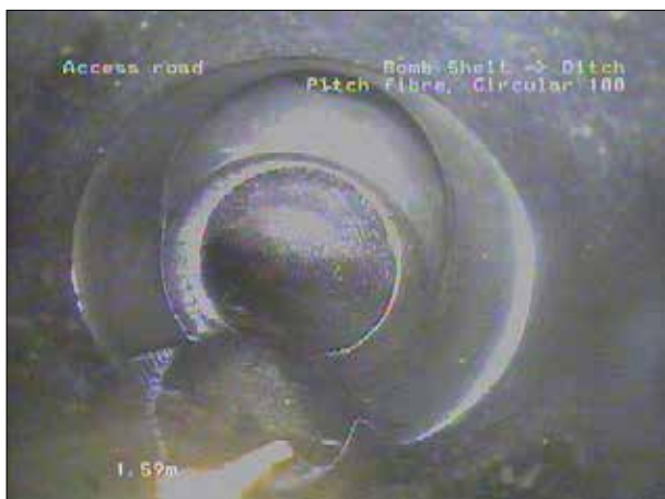
Photo: 31_4a, 00:00:00 1.59m, Junction at 12 o'clock dia 100 mm
