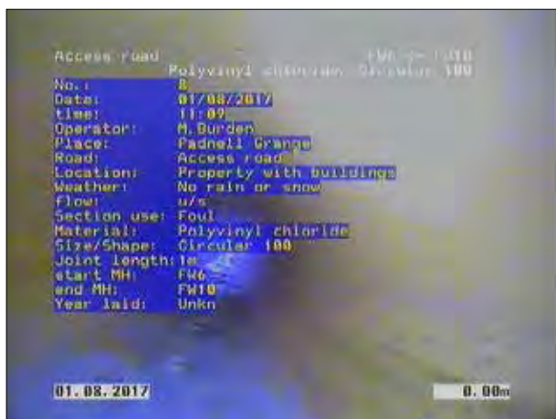
Photo: 55_1a 0m, Start node type, manhole, reference number: FW6
