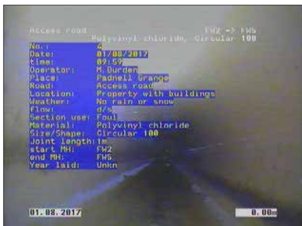
Photo: 4_1a 0m, Start node type, manhole, reference number: FW2
