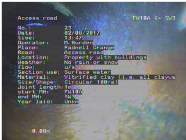
Photo: 170_1a, 00:00:00 0m, Start node type, manhole, reference number: FW10A
