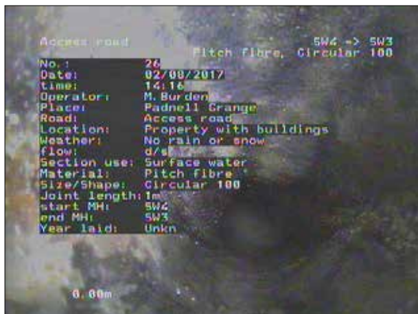
Photo: 188_1a, 00:00:00 0m, Start node type, manhole, reference number: SW4
