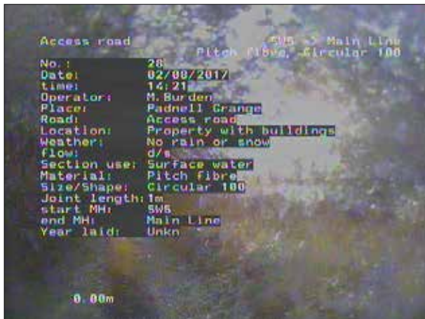
Photo: 30_1a, 00:00:00 0m, Start node type, manhole, reference number: SW5
