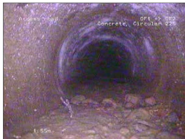
Photo: 120_4a, 00:00:00 1.55m, Survey abandoned, Remark: to much debris in line
