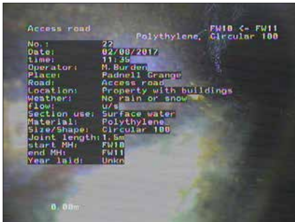
Photo: 159_1a, 00:00:00 0m, Start node type, manhole, reference number: FW10
