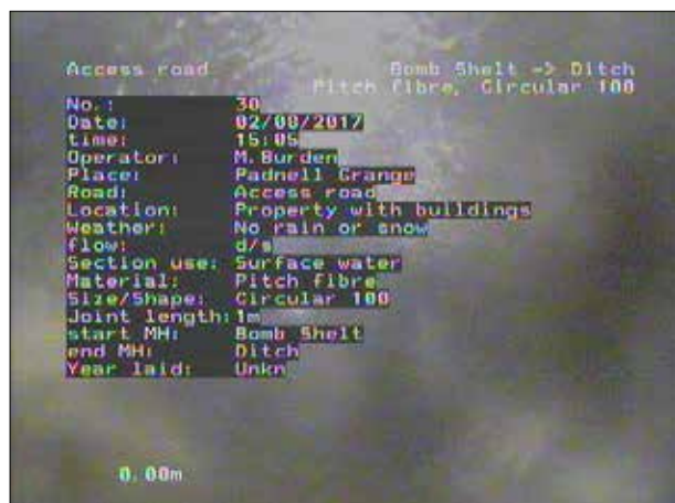
Photo: 210_1a, 00:00:00 0m, Start node type, manhole, reference number: Bomb Shelt
