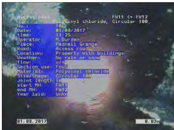
Photo: 61_1a 0m, Start node type, manhole, reference number: FW11
