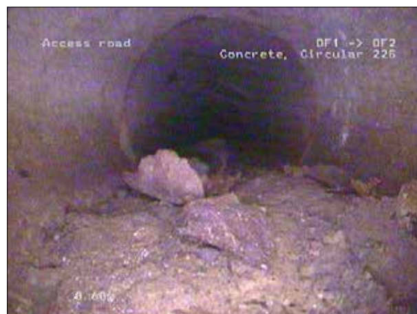
Photo: 118_2a, 00:00:00 0.6m, Settled deposits fine 10 % cross-sectional area loss
