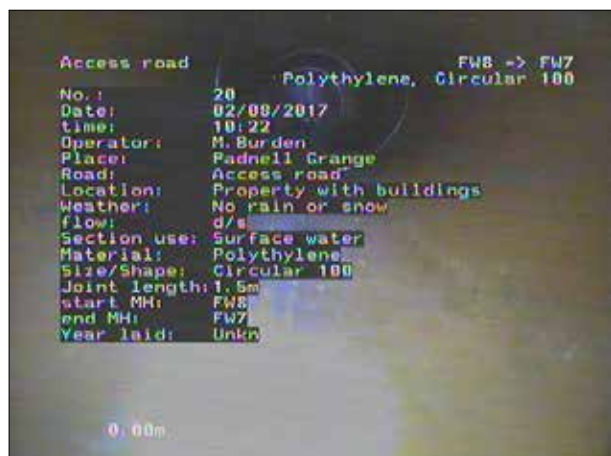
Photo: 132_1a, 00:00:00 0m, Start node type, manhole, reference number: FW8
