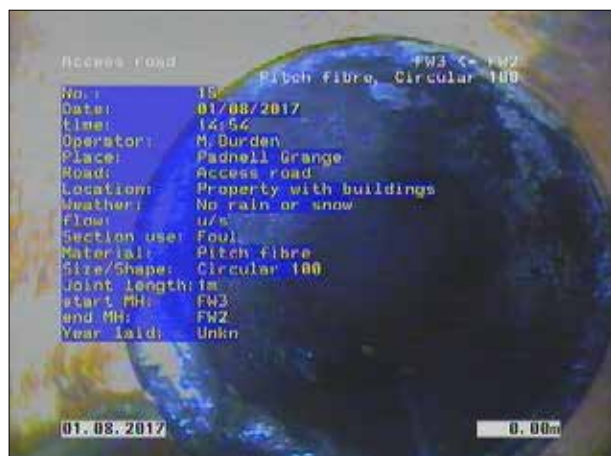
Photo: 101_1a 0m, Start node type, manhole, reference number: FW3
