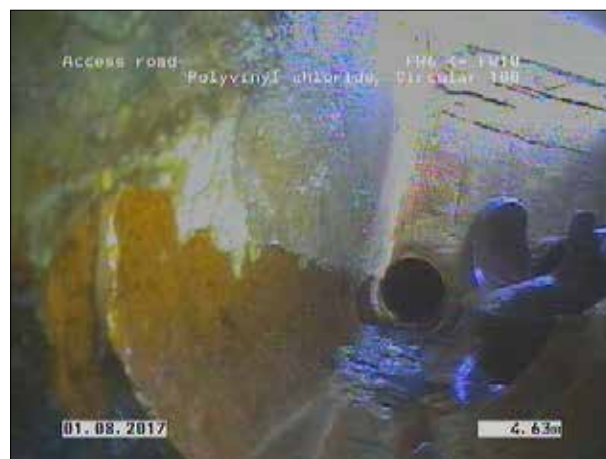
Photo: 57_3a 4.63m, Finish node type, manhole, reference number: FW10
