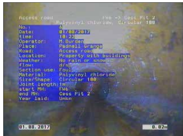
Photo: 6_2a 0m, Start node type, manhole, reference number: FW6
