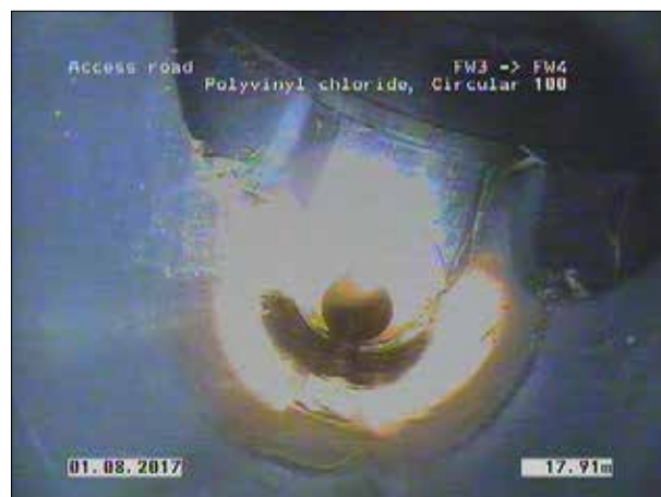
Photo: 108_3a 17.91m, Finish node type, manhole, reference number: FW4
