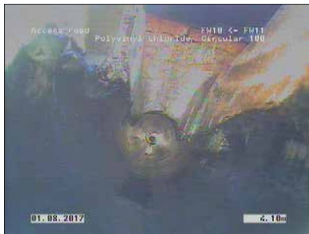
Photo: 60_3a 4.1m, Finish node type, manhole, reference number: FW11
