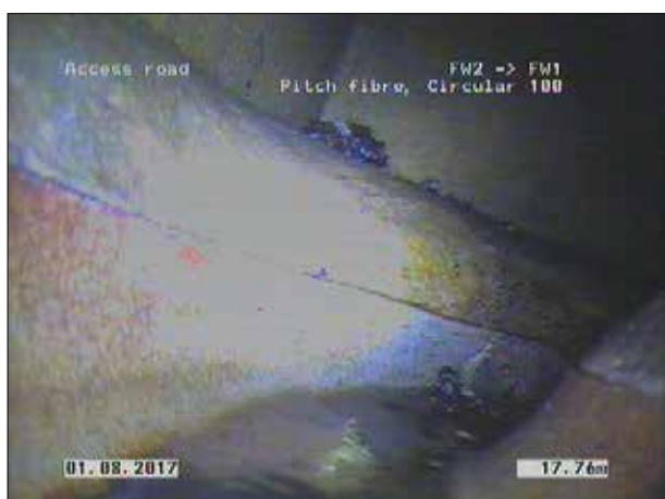
Photo: 3_16a 17.76m, Finish node type, manhole, reference number: FW1
