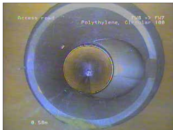
Photo: 134_3a, 00:00:00 0.56m, Junction at 03 o'clock dia 100 mm
