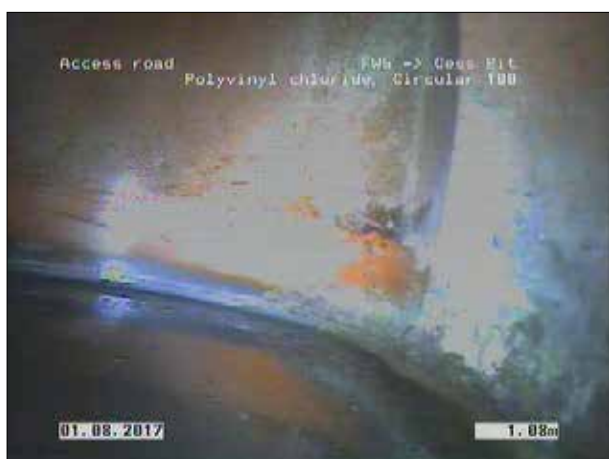
Photo: 44_4a 1.08m, Finish node type, other special chamber, reference number: Cess Pit
