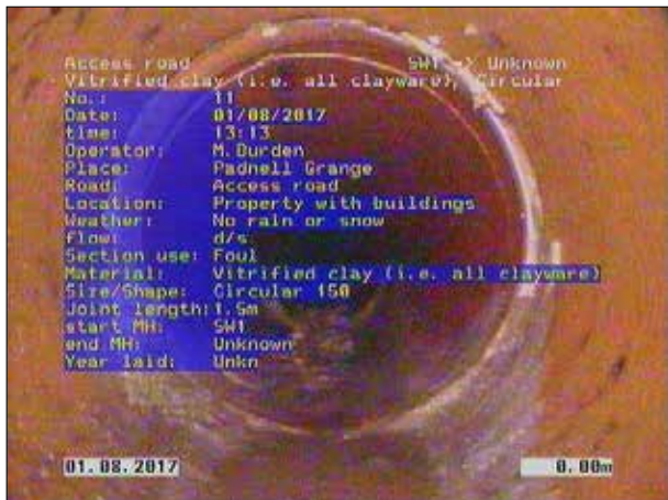
Photo: 64_1a 0m, Start node type, catchpit, reference number: SW1
