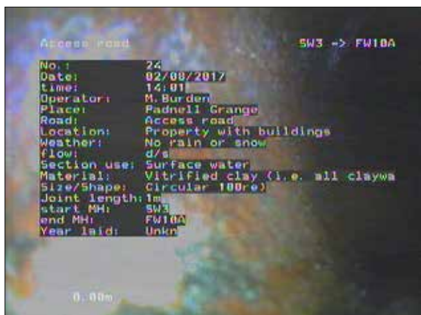
Photo: 177_1a, 00:00:00 0m, Start node type, manhole, reference number: SW3
