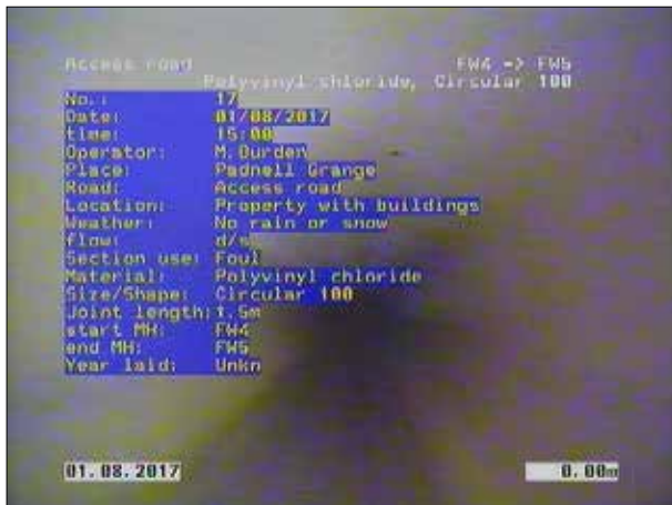
Photo: 109_1a 0m, Start node type, manhole, reference number: FW4
