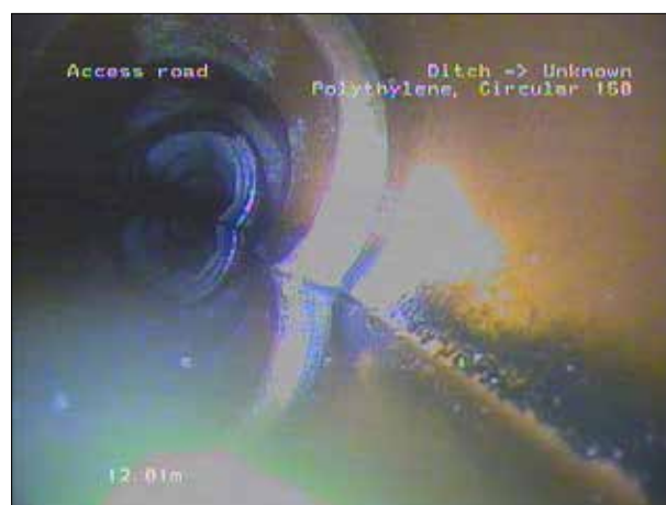
Photo: 226_5a, 00:00:00 12.01m, Material of drain/sewer changes to Vitrified clay (i.e. all clayware)
