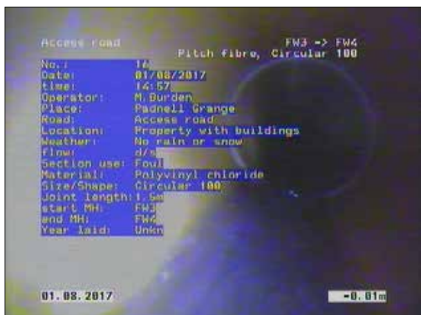
Photo: 106_1a 0m, Start node type, manhole, reference number: FW3
