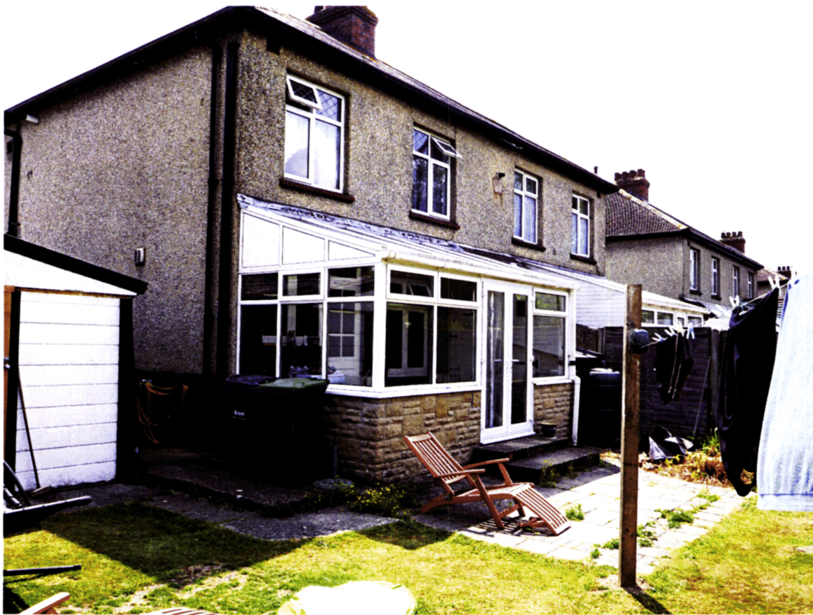
Rear view of 15 Elm Park Road
