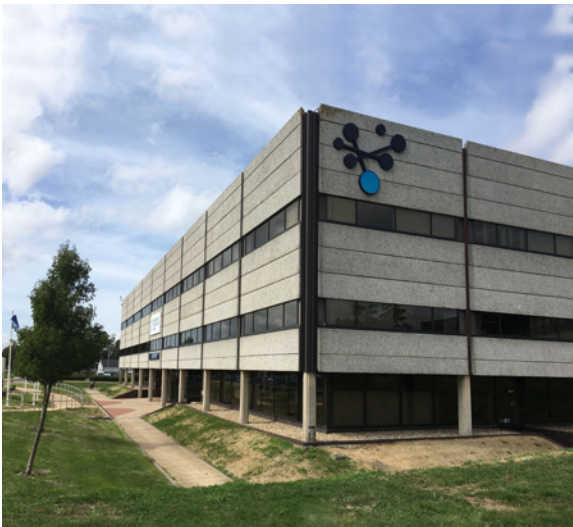
06 - Building 6000, south east corner.
