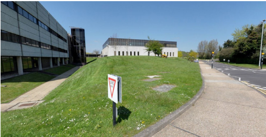
04 - Building 6000 (east elevation) concealed behind landscape bund.
