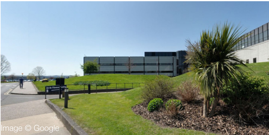
01 - East access, looking towards Building 6000. 7000 in the foreground.
