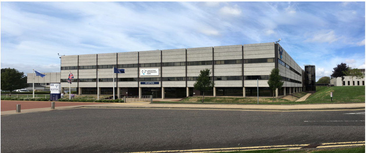
05 - Building 6000 south facade.
