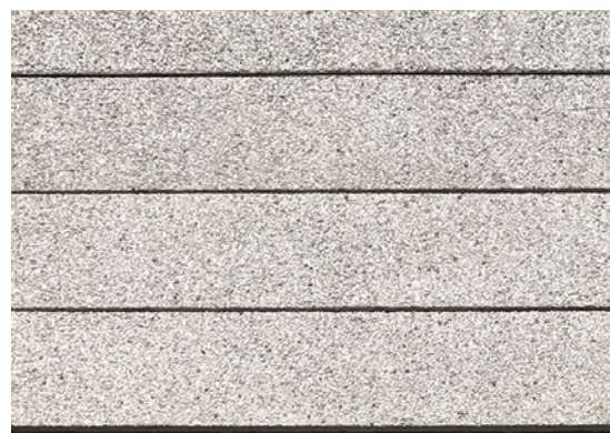
01 Pre-cast concrete panels - restored.
