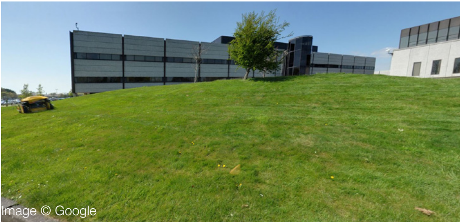
02 - Looking west, towards 6000. The east elevation is largely concealed.
