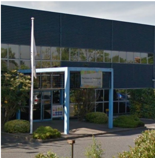
Existing office entrance and feature
