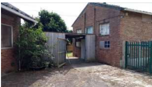
Photo 11. Northern elevation of B12.
