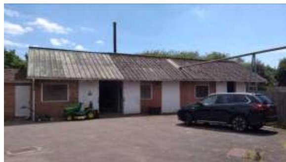
Photo 10. North-western elevation of B11.
