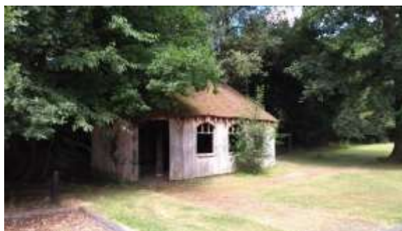
Photo 4. Eastern and southern elevations of B4.
