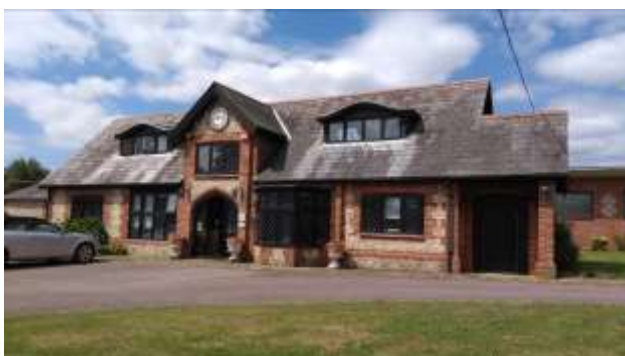
Photo 5. Eastern elevation of B5.
