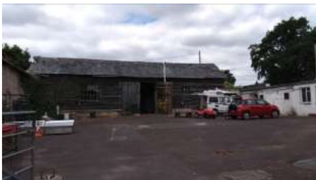
Photo 7. Eastern elevation of B7 and southern elevation of B6.
