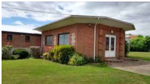
Photo 6. Northern and eastern elevations of B6.
