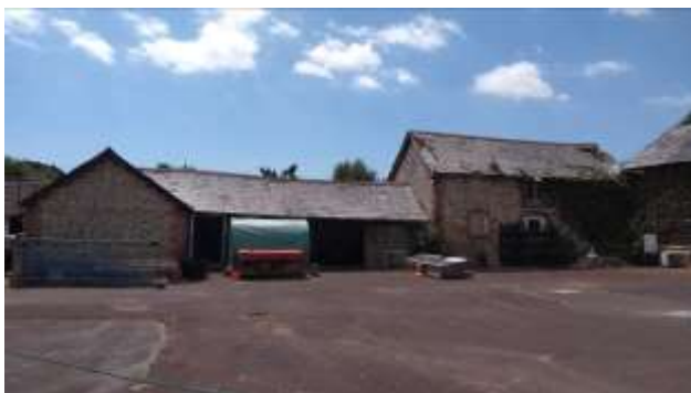
Photo 9. Northern elevation of B10.
