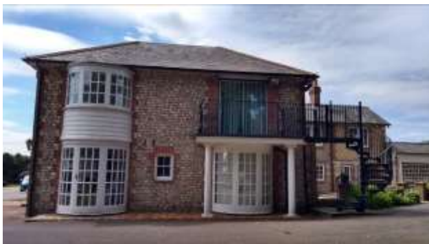
Photo 1. Eastern elevation of B1.
