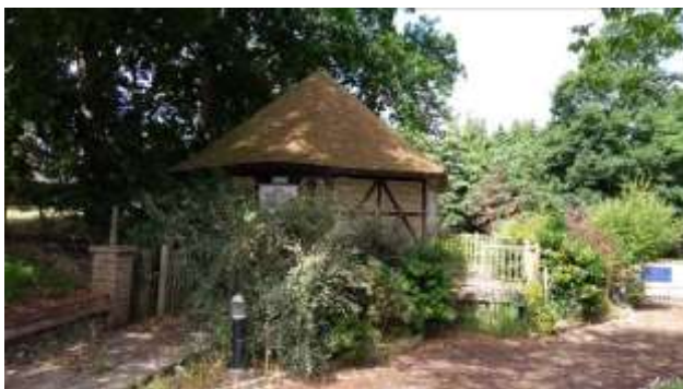
Photo 3. North-eastern elevation of B3.
