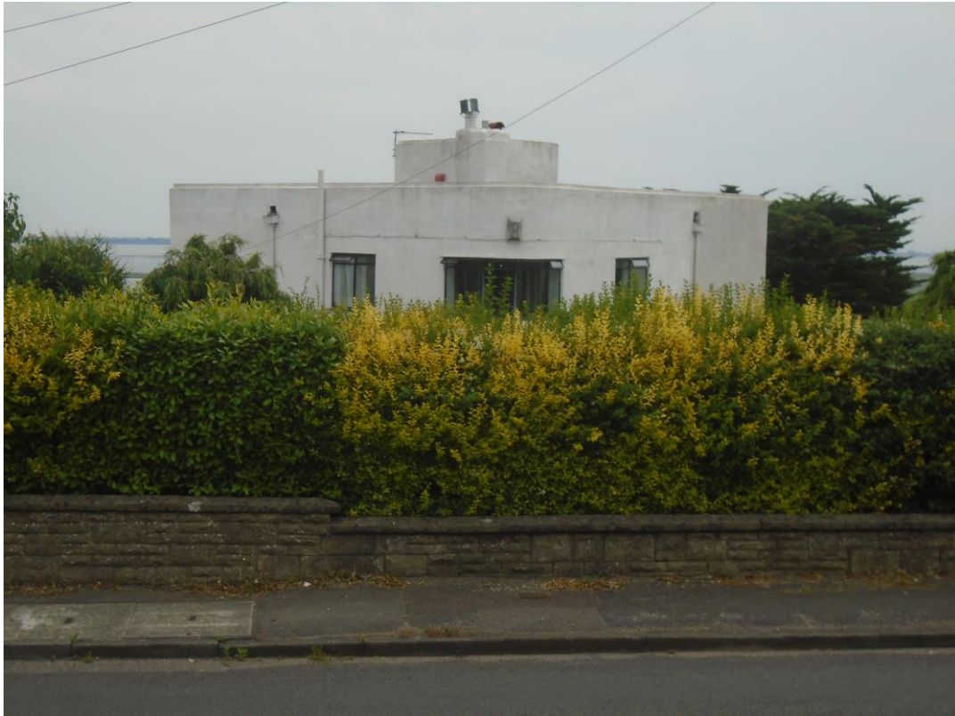
Figure 3. The frontage of Sunspan is largely screened by a mature hedge.
