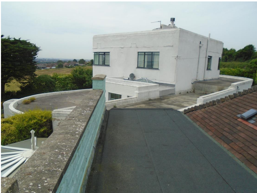
Figure 4. View from flat roof of No.47A looking towards Sunspan.
