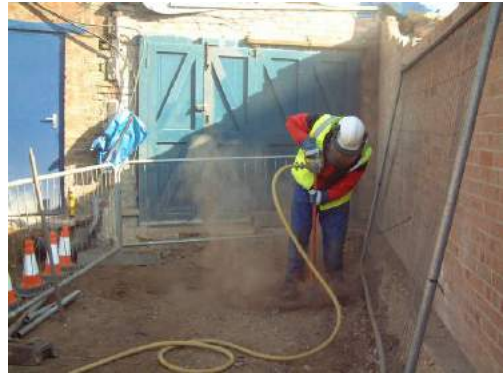
Photograph 2: Exposed undamaged roots following excavation with soil pick
