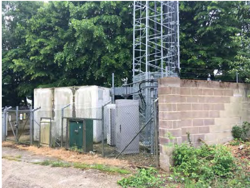
Photograph 4 – Radio mast and substation
