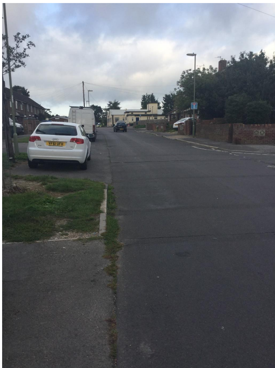
Fraser Road (junction with Woodgreen) west
