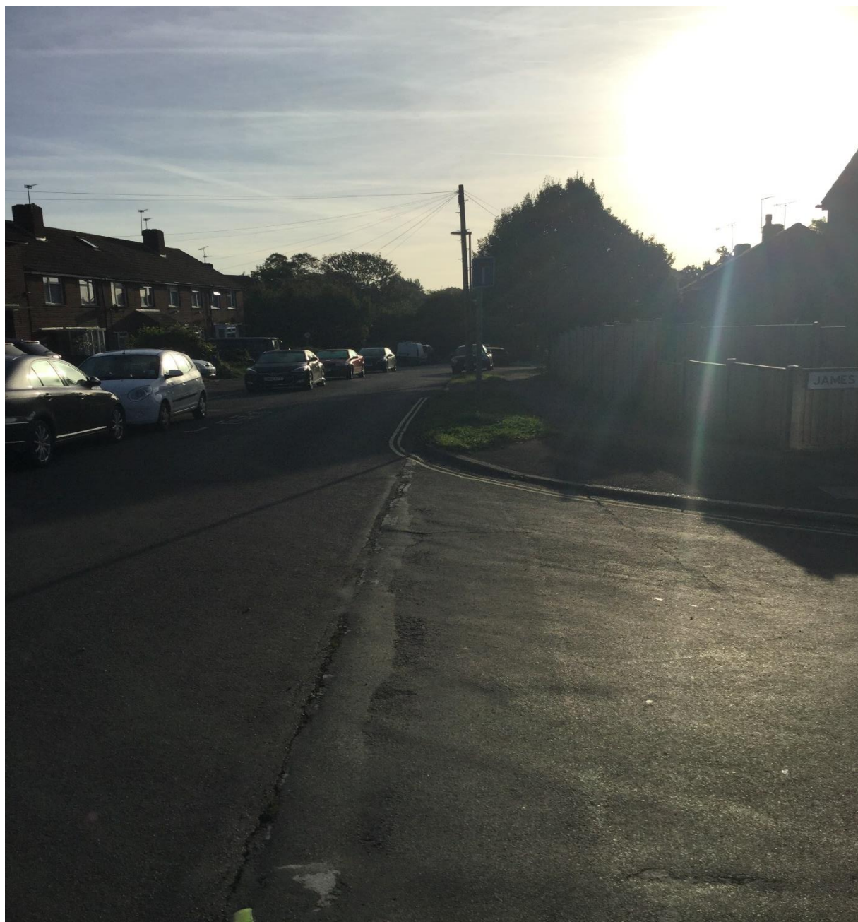
Fraser Road (junction with James Road) east
