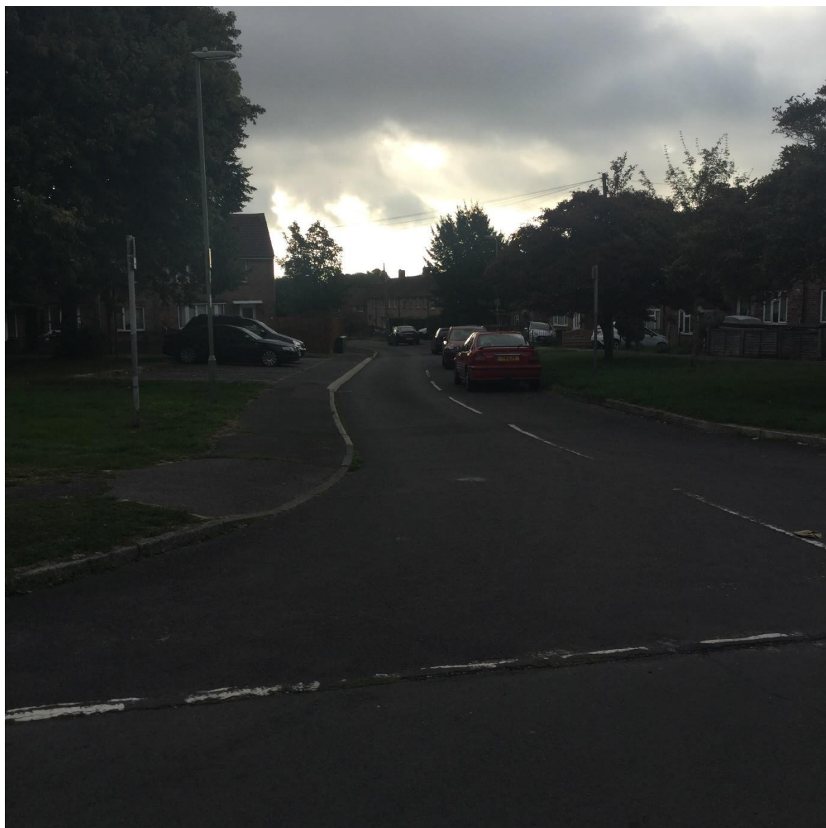
Woodgreen Avenue and Timsbury Crescent junction
