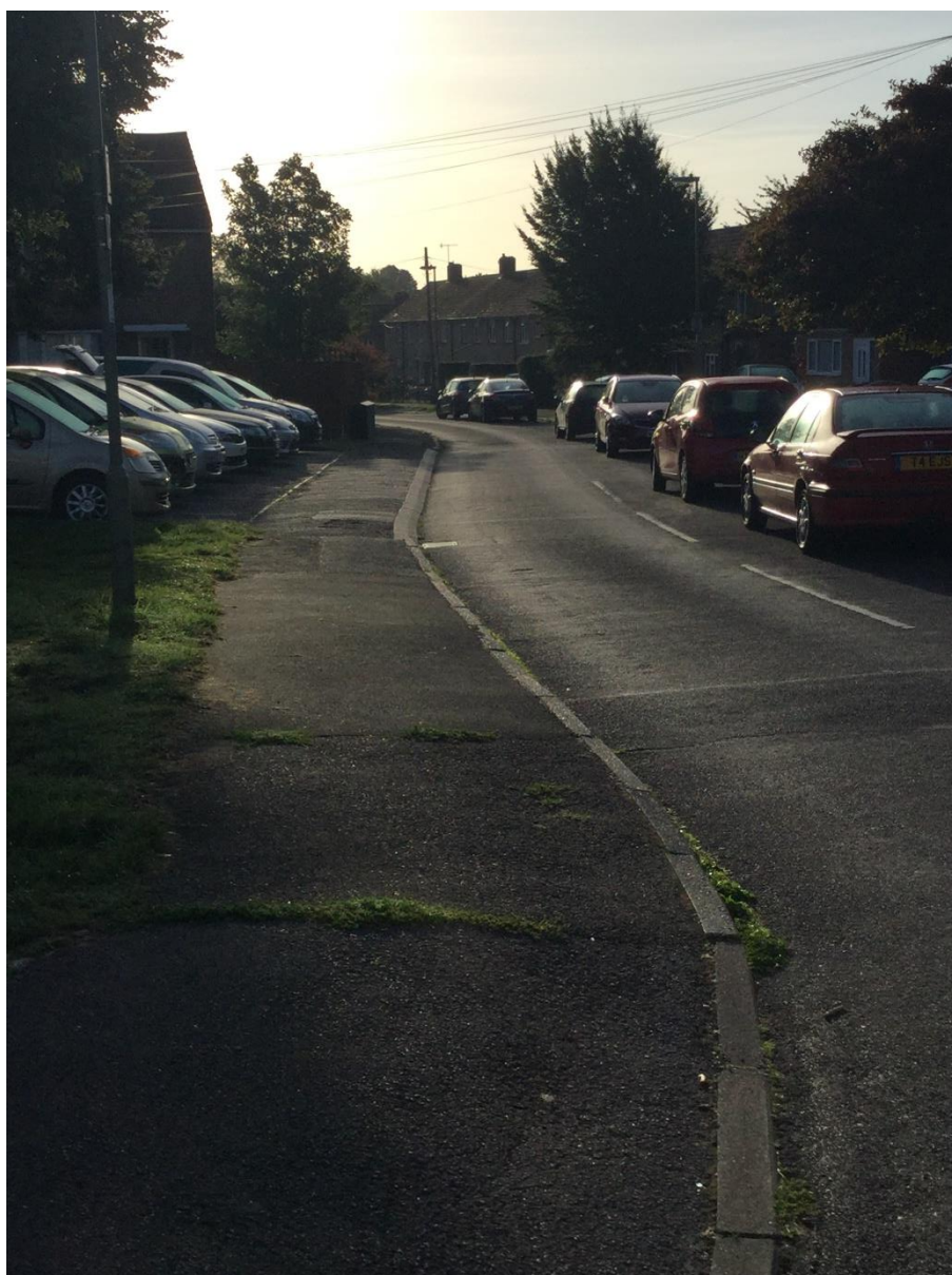
Woodgreen Avenue and Timsbury Crescent junction
