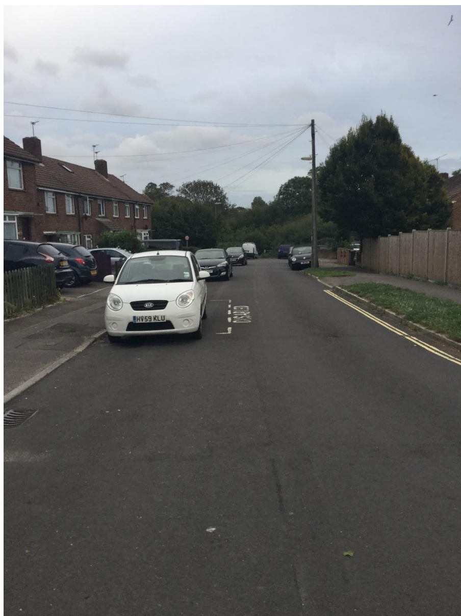
Fraser Road (junction with James Road) east
