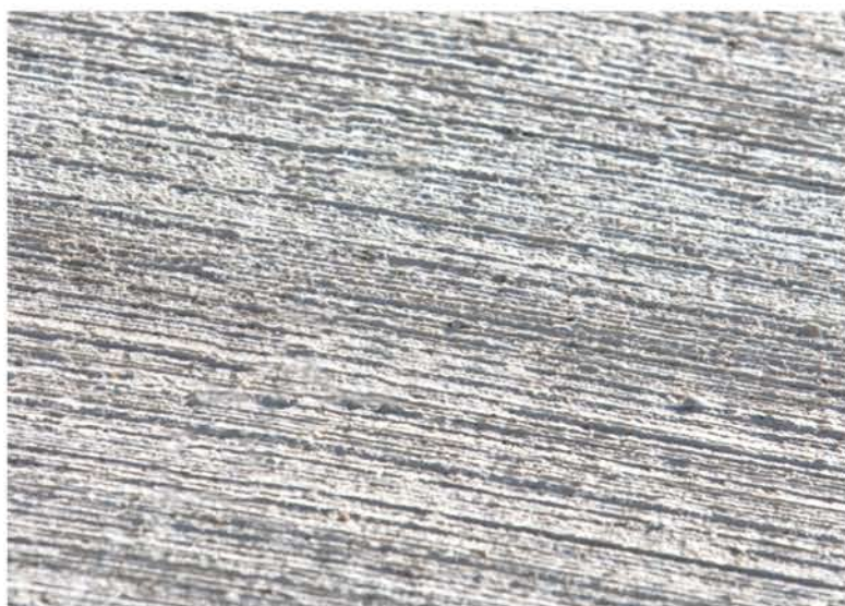
2. Brushed concrete hardstand
