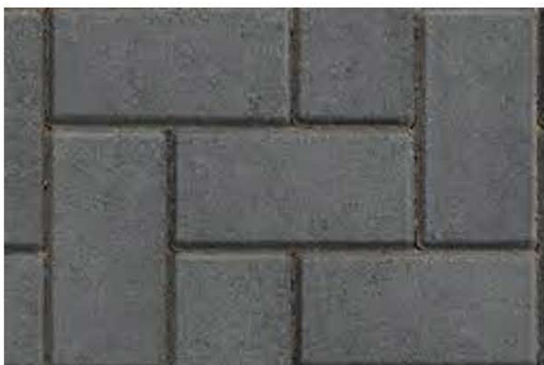
3. Keylock concrete block paving
