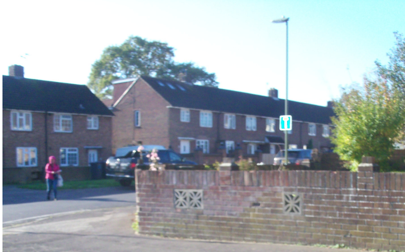
Properties on Fraser Road adjacent to the application site
