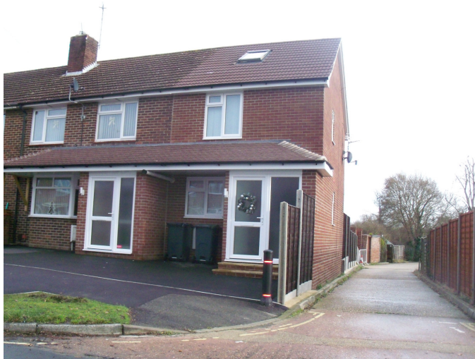
Example infill residential development at 7A James Road
