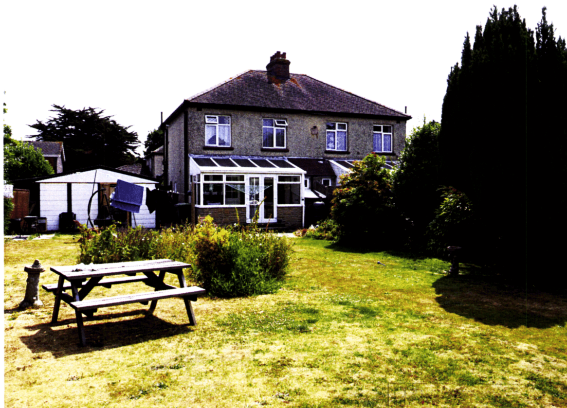
Rear elevation and garden to 15 Elm Park Road
