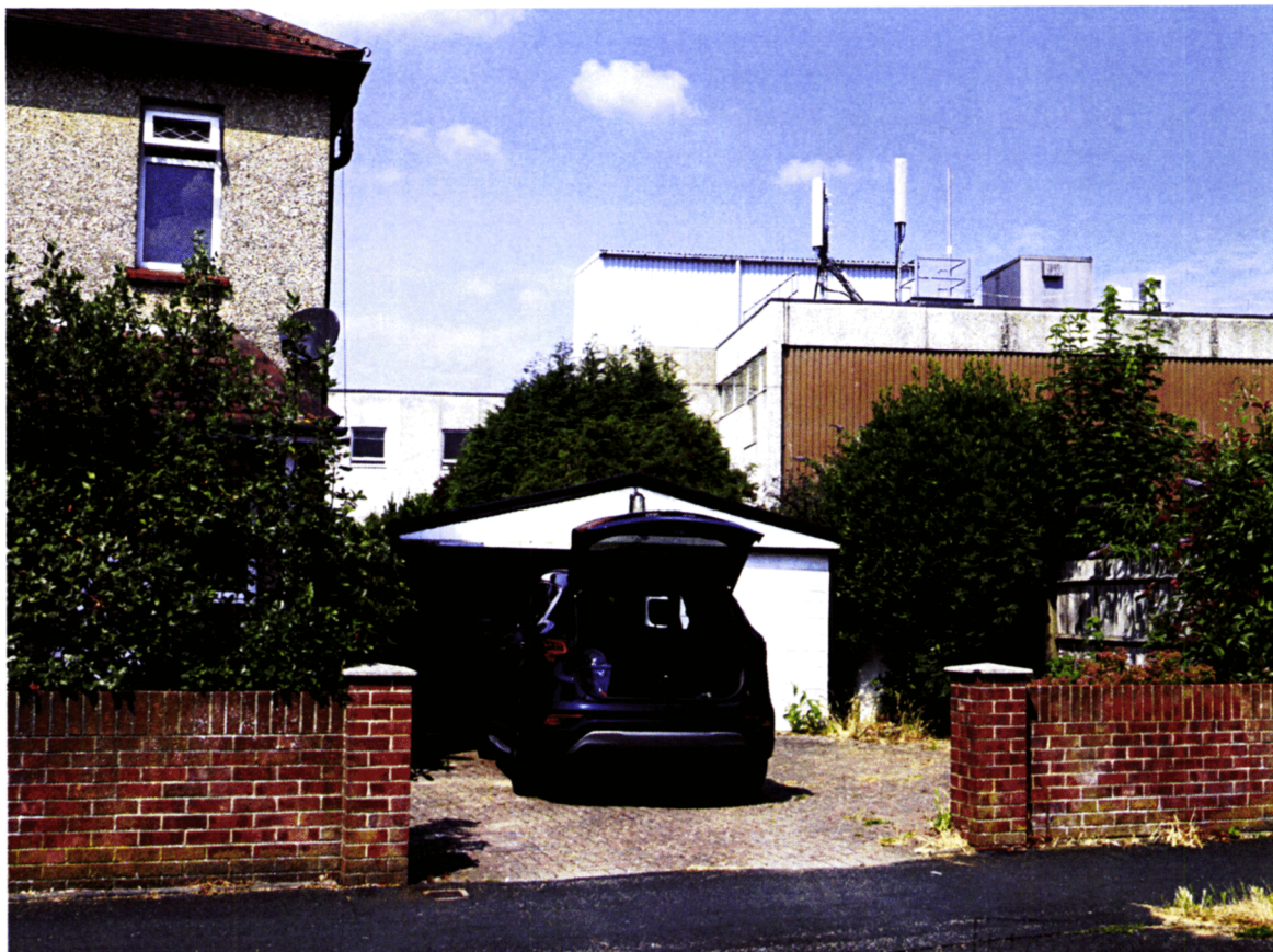
Existing vehicular access and garage to 15 Elm Park Road
