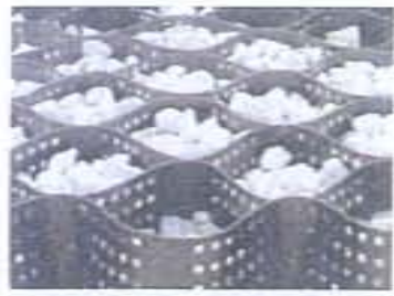
Cellweb TRP access road during filling with clean stone.
