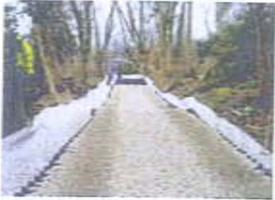
Cellweb TRP access road during filling with clean stone.
