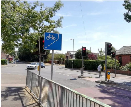
Photograph 65: Signal Control Crossing at Emsworth Road
