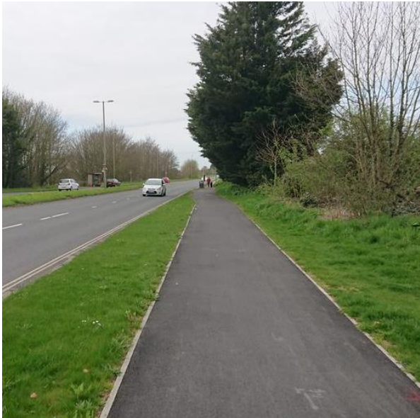
Photograph 2: New footway/cycleway along Havant Road
