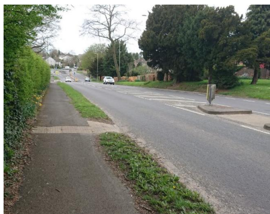
Photograph 47: Footway Conditions along Bedhampton Road
