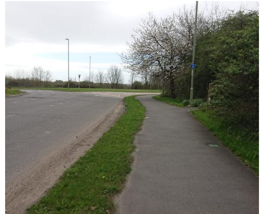
Photograph 5: Footway/cycleway on Rusty Cutter leading up to A3M northbound on-slip
