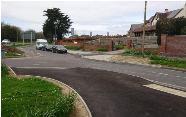
Photograph 4: Where cyclists re-join footway/cycleway
