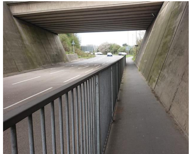
Photograph 7: Footway under A3M Motorway Bridge
