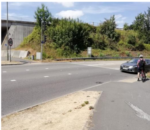
Photograph 8: Crossing across A3(M) southbound
