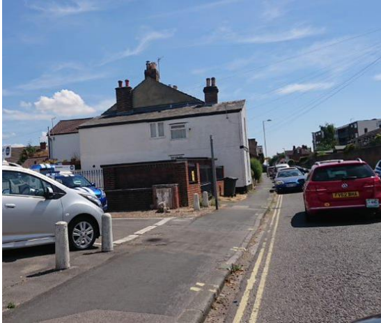
Photograph 61: Conditions along West Street
