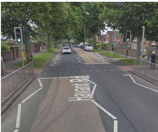
Photograph 79: Signal control crossing adjacent to Portsdown Avenue
