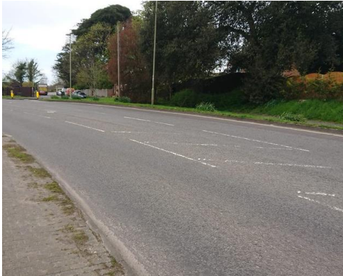
Photograph 12: Location of existing hatching and new pedestrian refuge island
