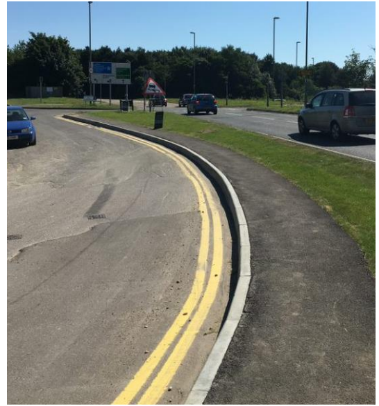
Photograph 3: Footway on Bedhampton Hill (Where footway/cycleway ceases)
