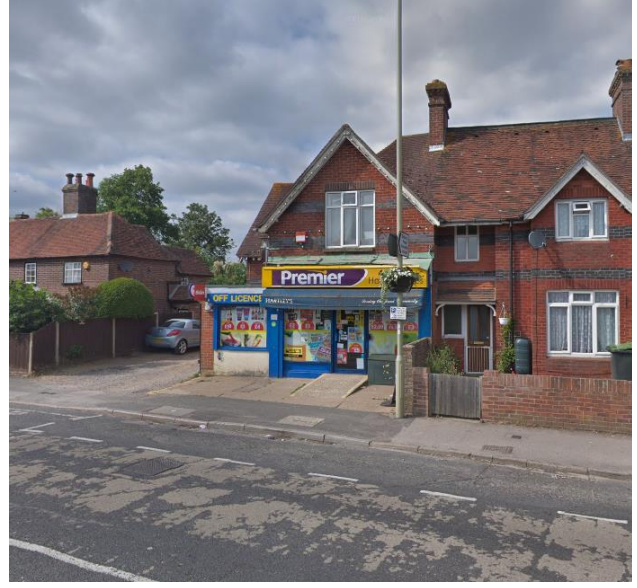
Photograph 39: Footway along Bedhampton Road (east of signalised junction)
