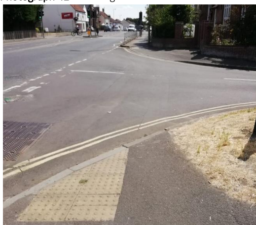
Photograph 44: Crossing at Kings Croft Lane
