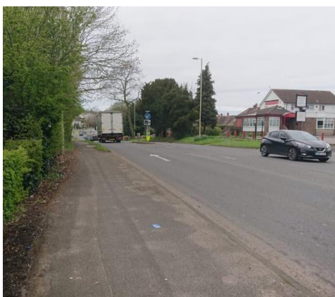
Photograph 46: Footway Conditions along Bedhampton Road
