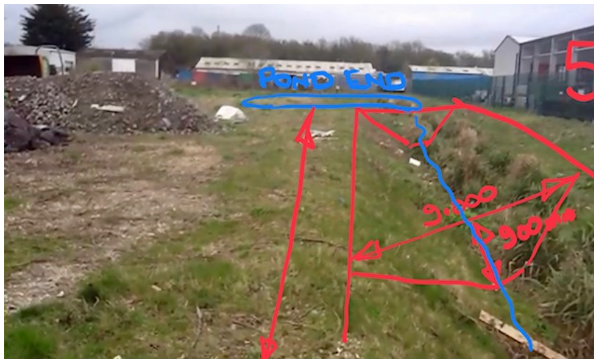
Ditch/swale looking east from service road culvert.
