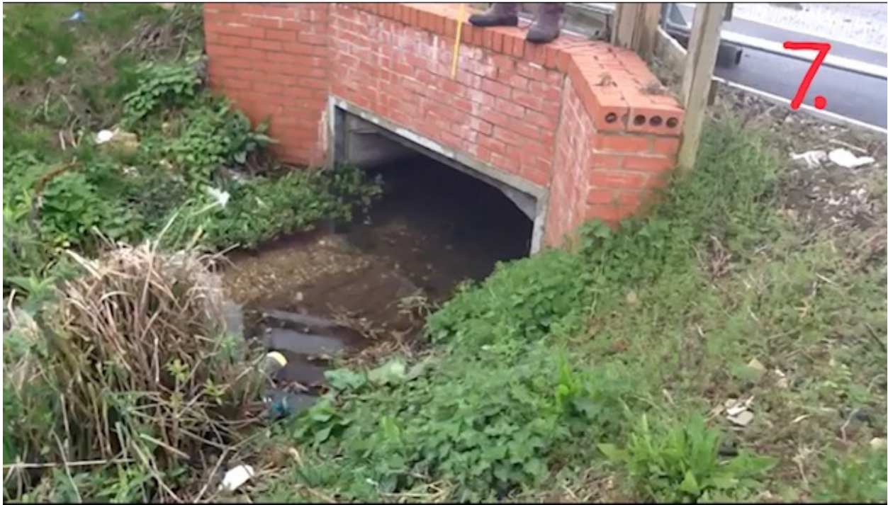
7. Culvert under service road
