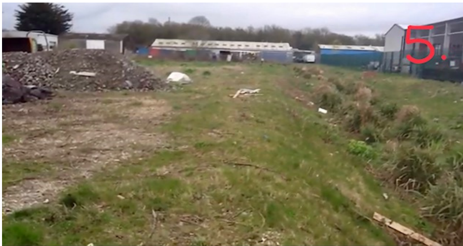
4. Running ditch from pond from service road culvert looking east towards pond.
