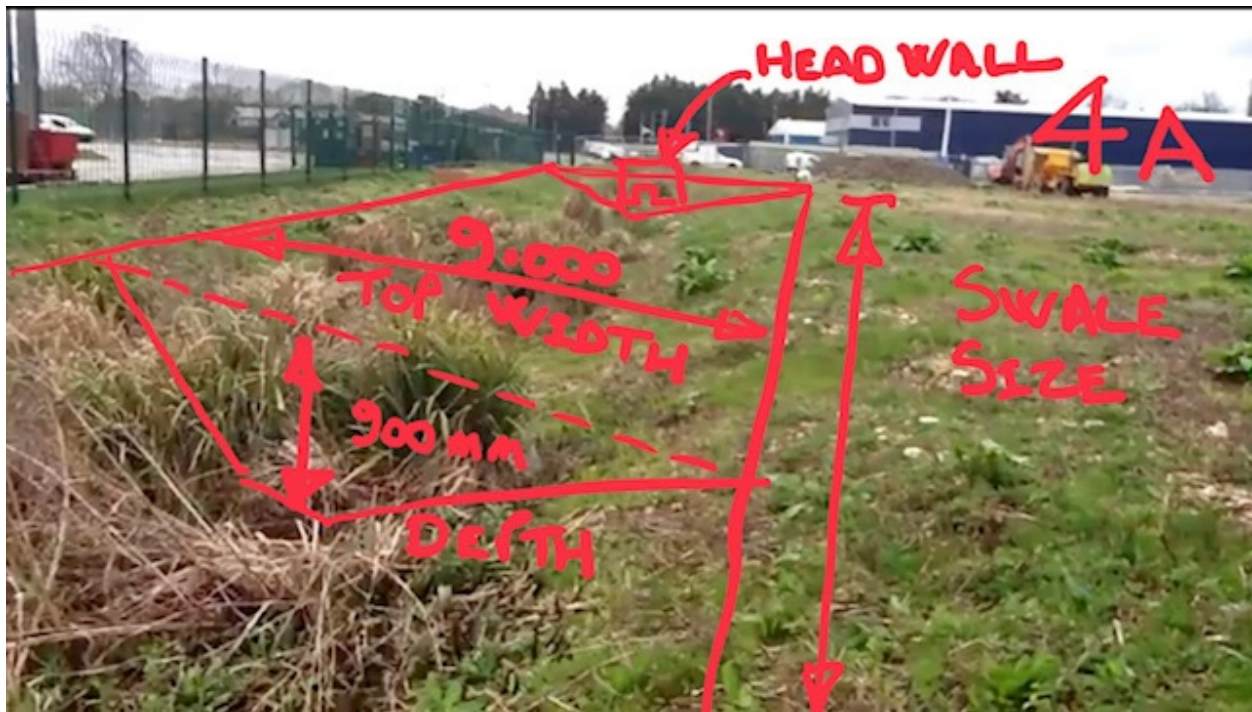
Ditch/swale looking west from southern end of pond.
