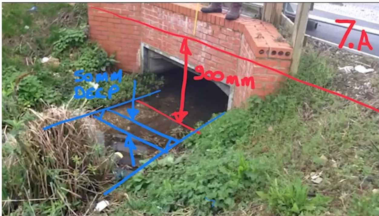
Culvert under service road indicating constant depth of water and water brake.
