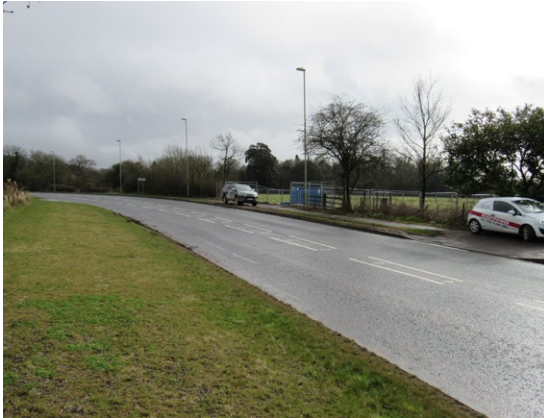
Approved access location looking east on Bartons Road
