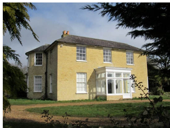
Grade II Listed East Leigh House on northern boundary
