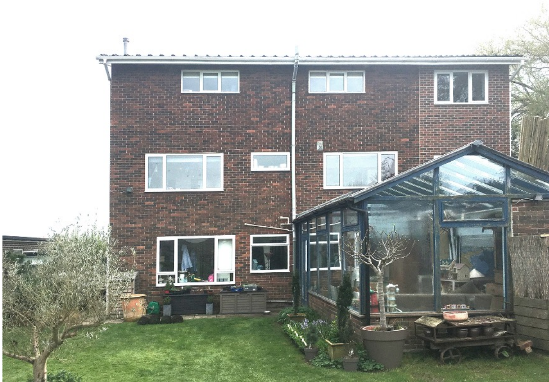
Photograph of existing rear elevation.
