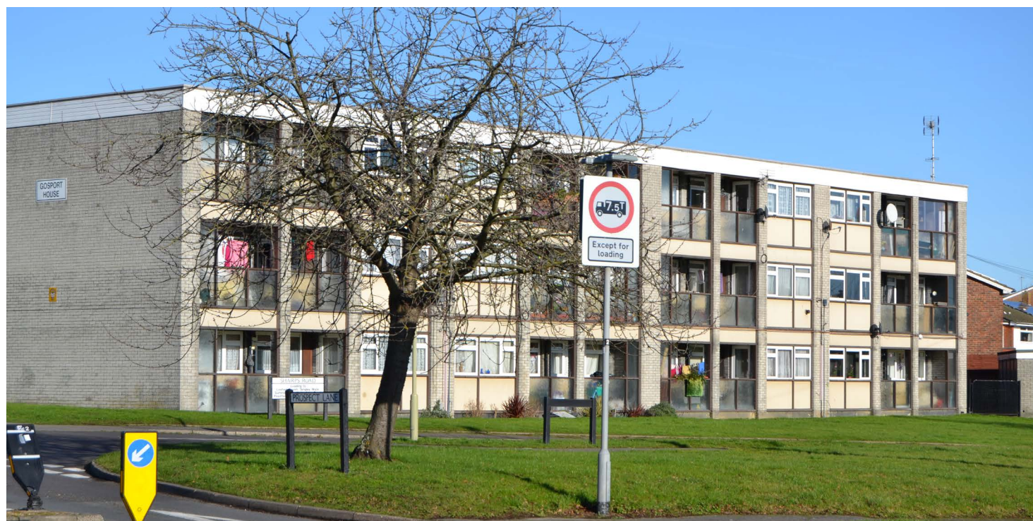
The flats to the north of the site, visible from Bartons Road.
