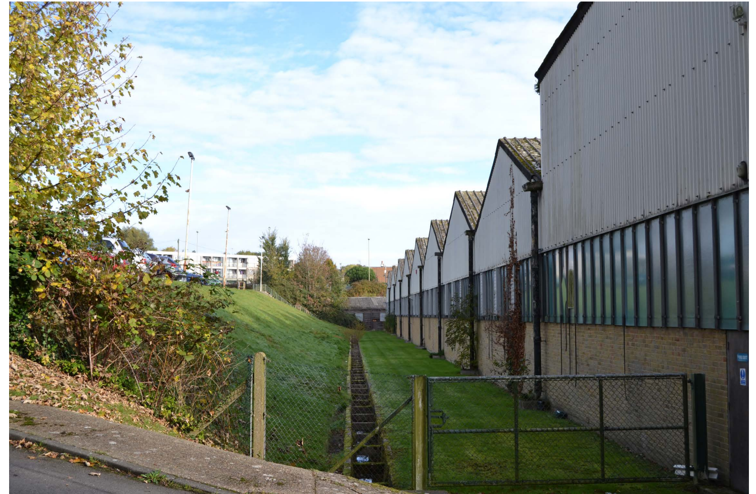
An image of the culvert in it's current undeveloped state.
