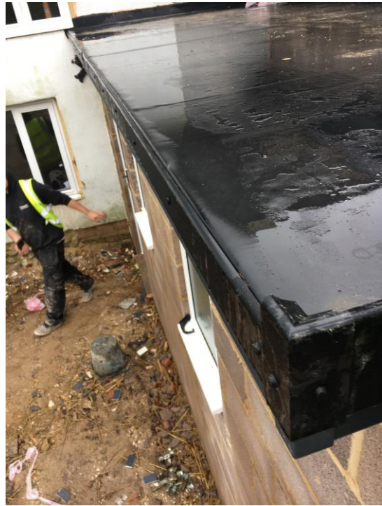
Main building roof Firestone EPDM
