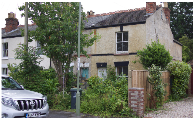
Fig (4) Repositioning of street-light
