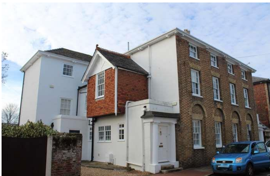
(Fig.3 Main facade facing King Street)
