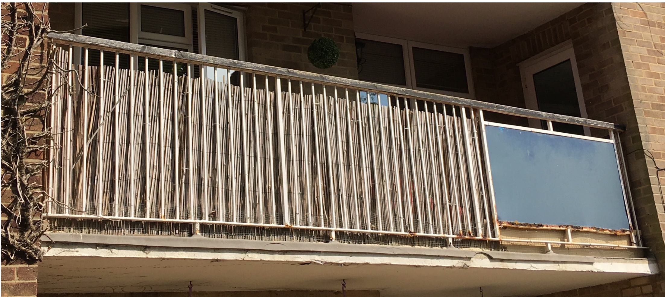
PICTURES OF THE EXISTING BALCONIES
