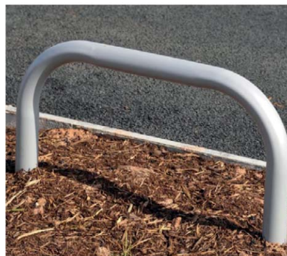
Hooped tubular rail to boundary of display parking spaces and entrance
