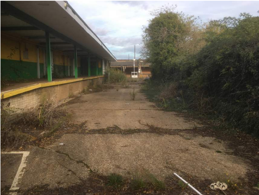
Plate 3. View looking into the central portion of the site from Dunsbury Way, with Co-operative funeral care to the right the other side of the hedge (2018).
