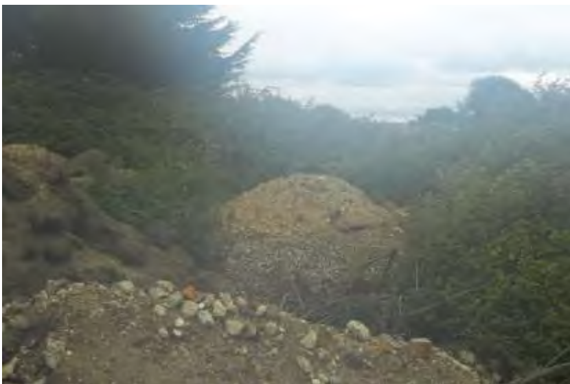
Stockpiles of earth and demolition spoil in south eastern part of site.
