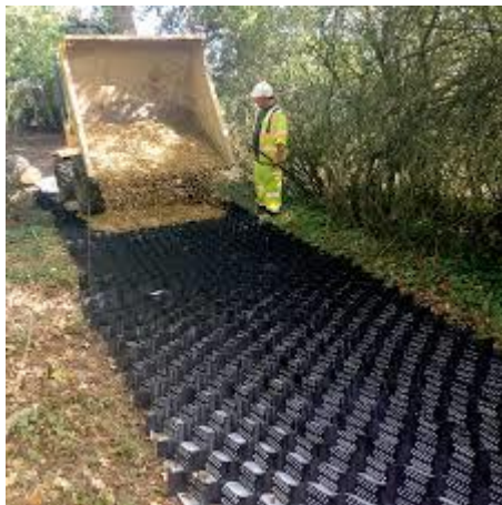
Photo shows Cell-web in situ being back filled.
