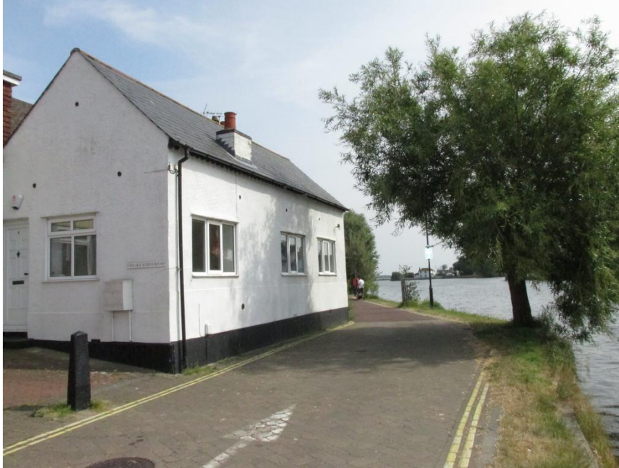
Figure 3: View from Bridgefoot Path looking south
