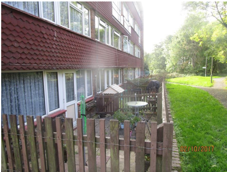
Photo 4 - Tile hanging to front elevation and existing boundary fencing.
