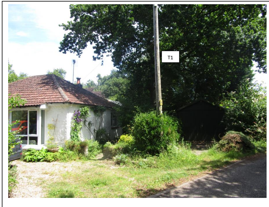
View of front right corner of dwelling
