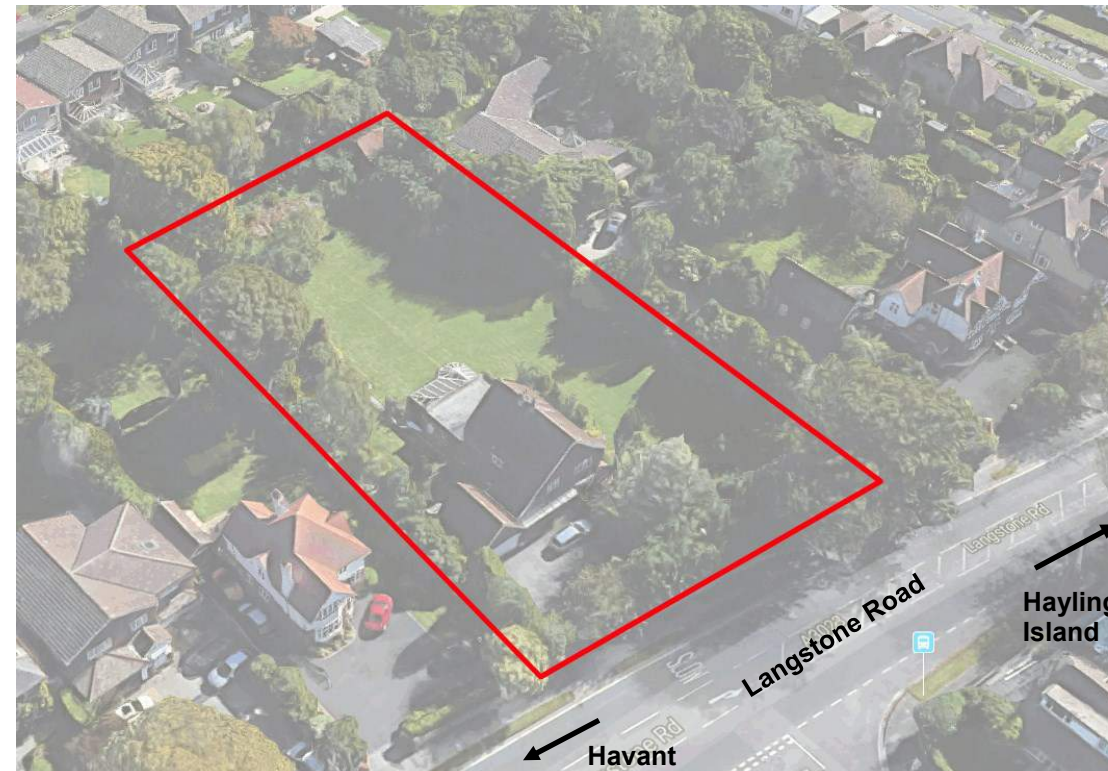
01 | Aerial view of the site (courtesy of Google Earth)
