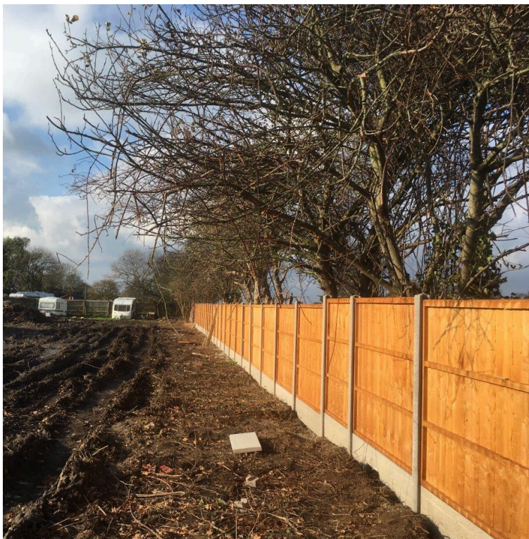
Figure 6. Defunct hedgerow running along the northern boundary with dry ditch in adjacent arable field.
