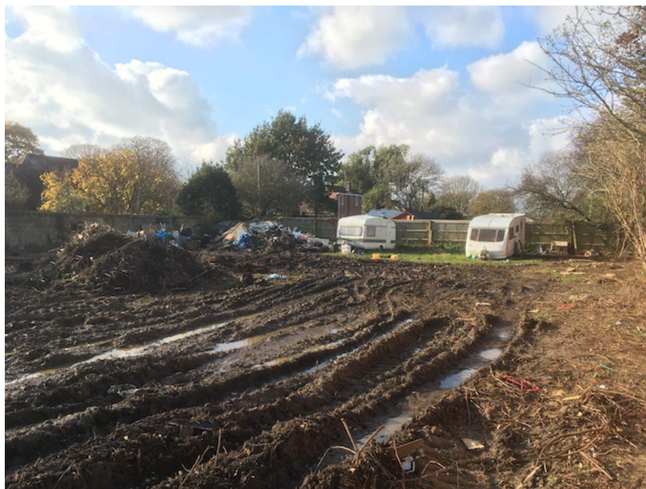
Figure 3. Bare ground on site with waste piles from site clearance.
