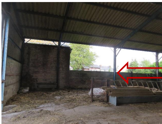
Interior of Barn (1 st Two Bays Removed)
