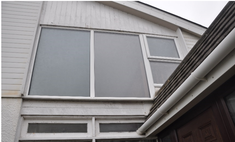
Figure 17: Current east facing first floor windows
