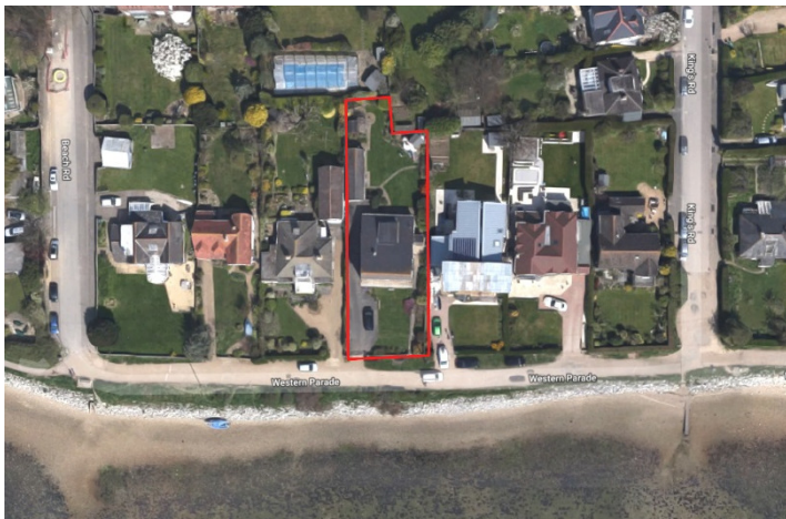
Figure 1: Aerial View of existing site
