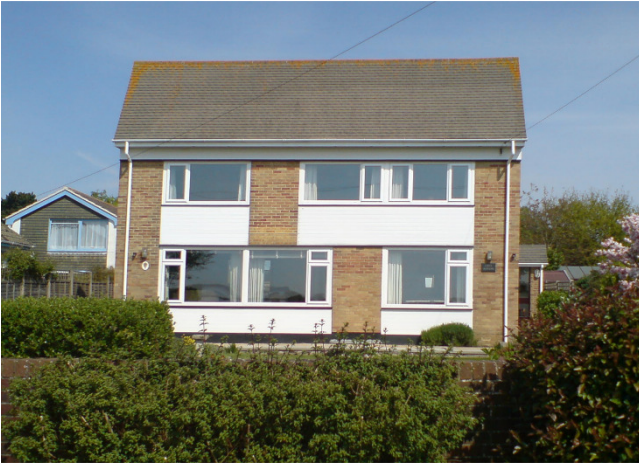
Figure 3: South elevation of existing building
