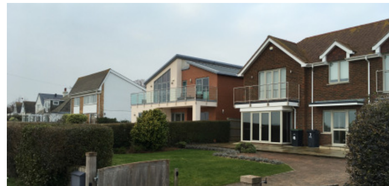
Figure 8: No.9 is the only building on Western Parade to have a skewed gable and is an anomaly on its road
