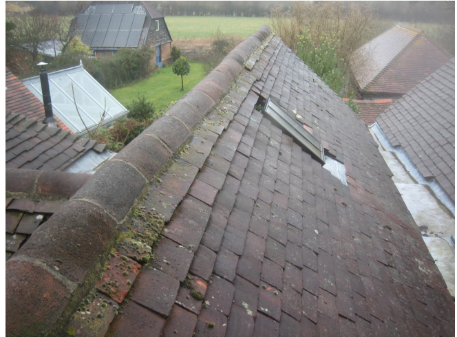
Fig 2 – photo of existing roof tiles
